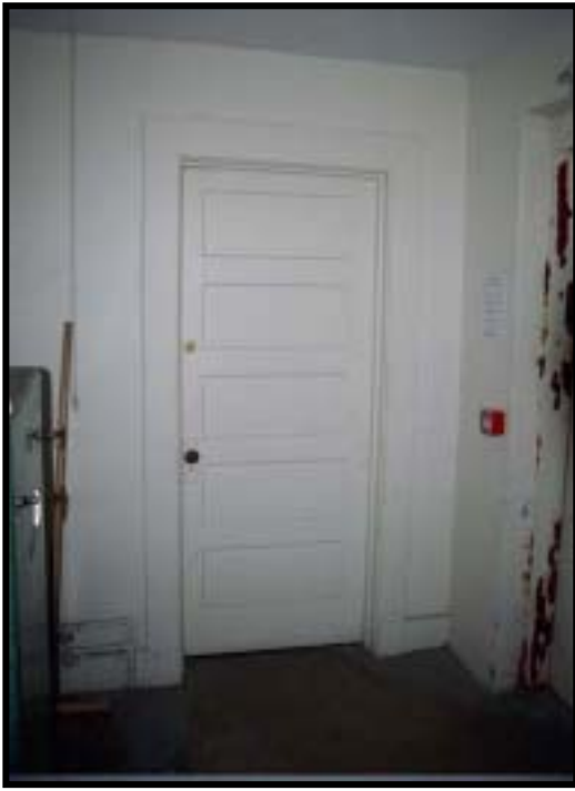
Figure 33. Original five- panel door located in northwest corner of kitchen.
