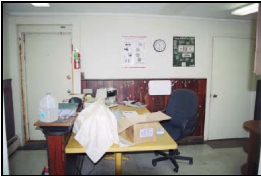
Figure 23. East wall of room 101, showing original east exterior doorway, D-101 (left), and added doorway to annex/watchtower, D-104 (right).
