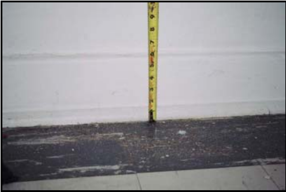
Figure 31. Original baseboard found on north wall of room 104.
