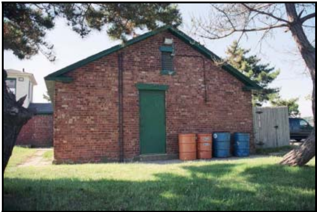
Figure 19 (below). North gable-end wall of main building of Gatehouse.
