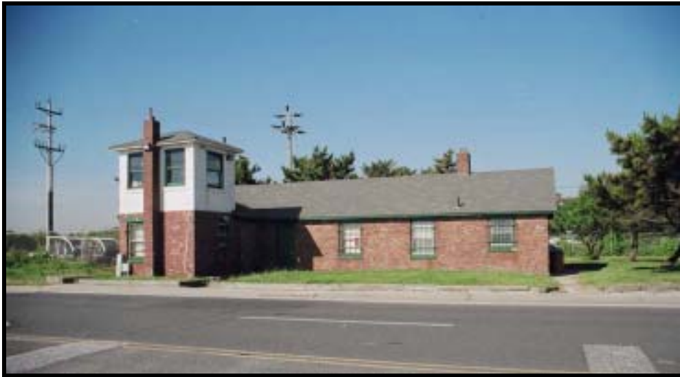
Figure 16. East elevation of Gatehouse.
