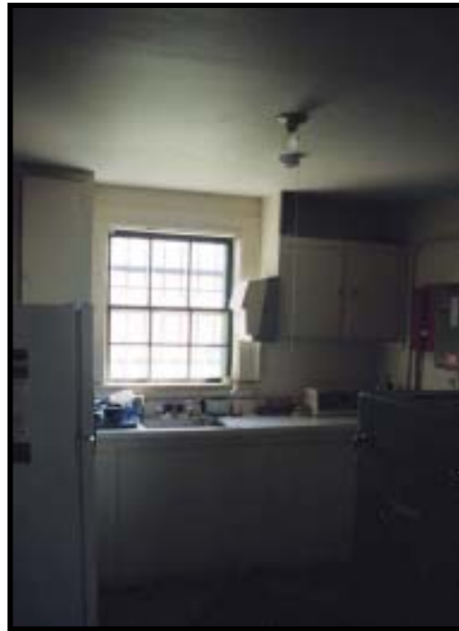
Figure 34. View of east wall of kitchen.
