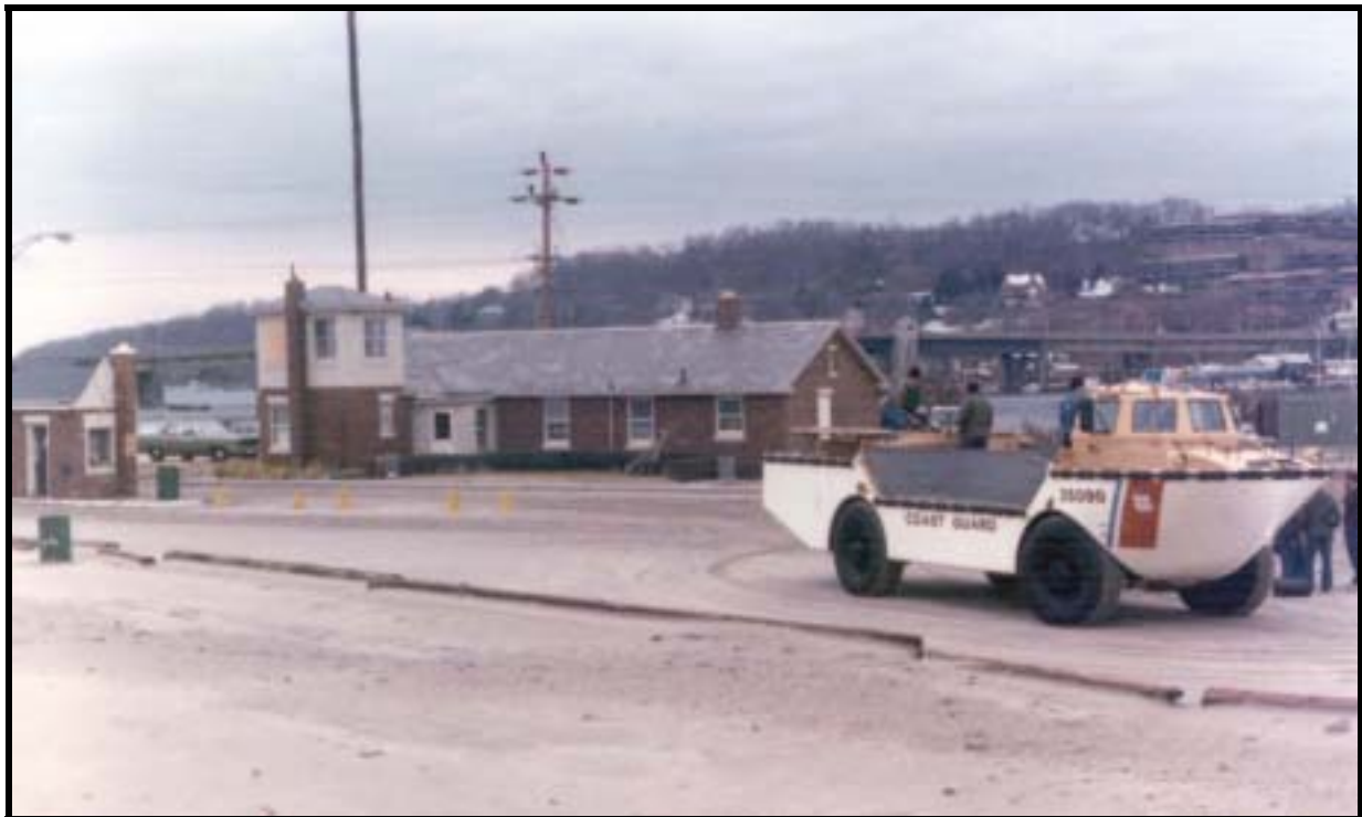
Figure 9. Fort Hancock Gatehouse ca. 1974- 75, showing wood- framed entrance vestibule added to the building about this time.
