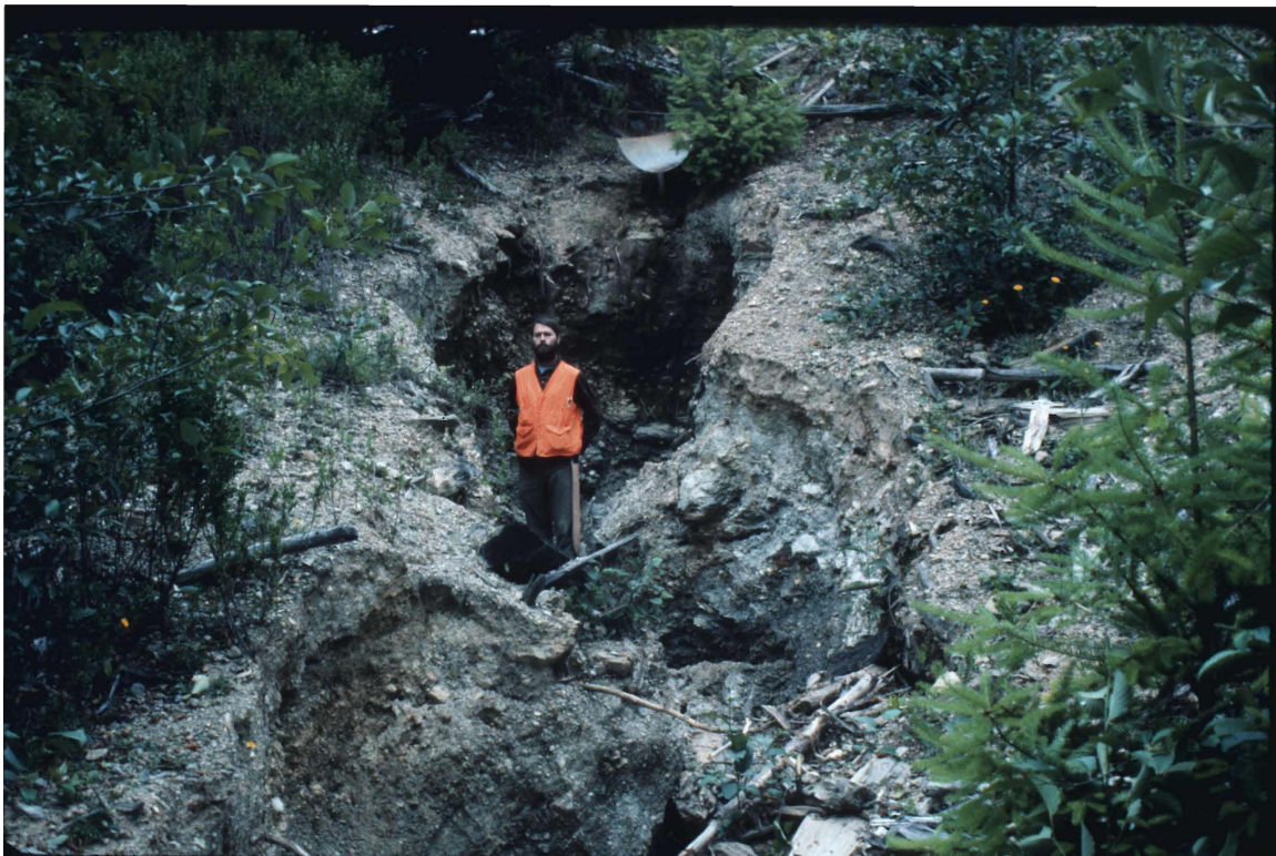
Unit: 80-6 PP#7 Gully at culvert outlet, Pre H.E. 1980
