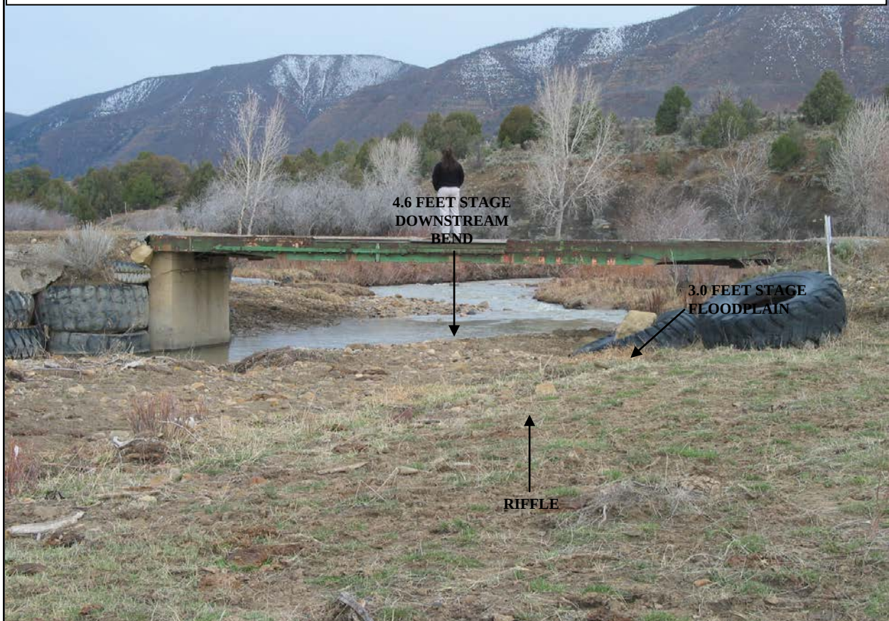
Figure 4: Looking downstream at Mancos River at Anitas Flat Station channel controls. Photograph taken April 9, 2006 by Gwen Gerber
