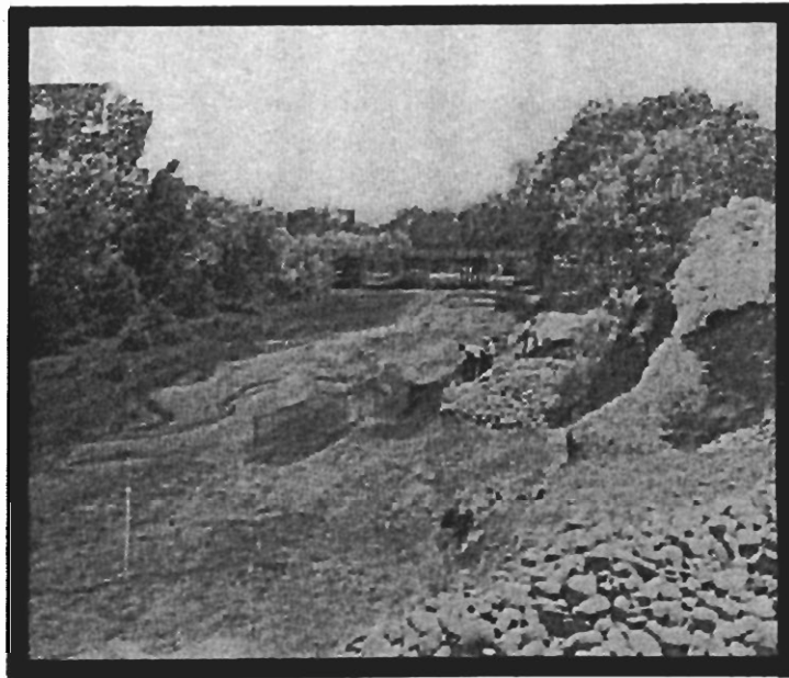
Photo 11: Construction of a gabion to provide bank stabilization at Wide Reed Ruins (20 July 1974), view to the northeast, highway bridge upstream.
