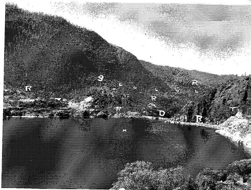
Fig. 46. Vicinity of O'Shaughnessy Dam, showing roads (R), tunnel (T), motor boat (M) one of the steel towers supporting the tramway (S), the tramway (L), and other developments. D — the dam itself, which is being raised an additional 85 feet.
