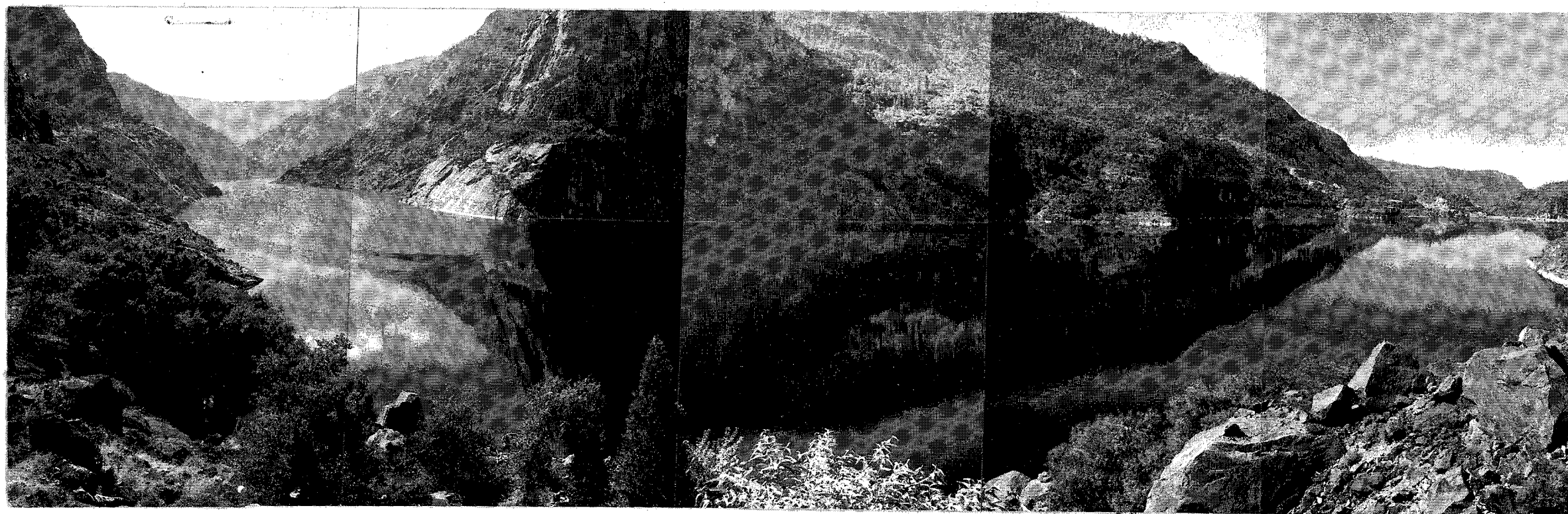
Fig. 45. Hetch Hetchy Reservoir as seen from opposite Kolana Rock. The dotted line indicates a previous water level; when the present construction is completed, the level will be 85 feet higher yet. K- Kolana Rock; D- O'Shaughnessy Dam; E- excavation in side of mountain to obtain rock for cement work.
