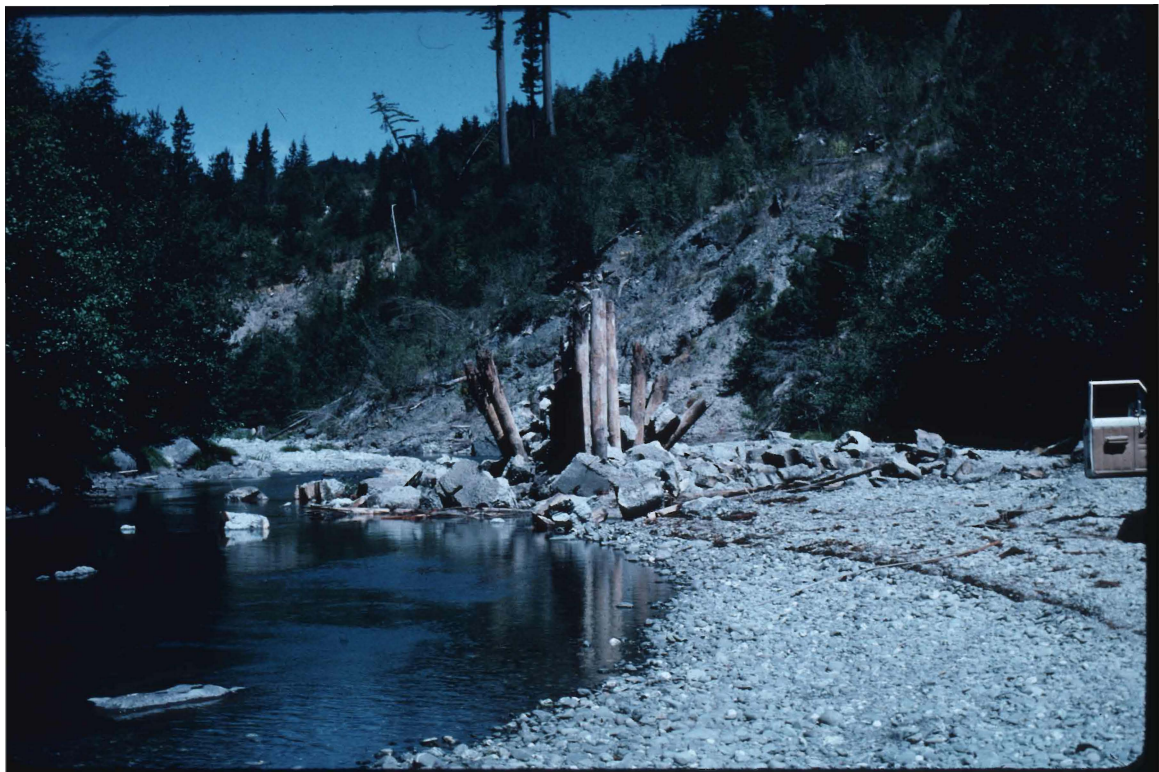
Unit: 84-3 1800 Rd. Redwood Cr. Bridge Site. Fall 84
