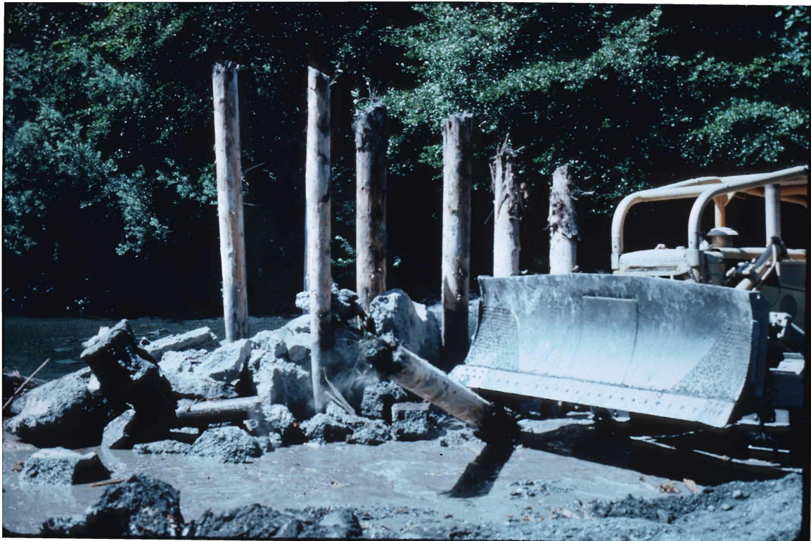
Unit: 84-3 Redwood Cr. Old1800 Rd. Bridge pilings Fall 84
