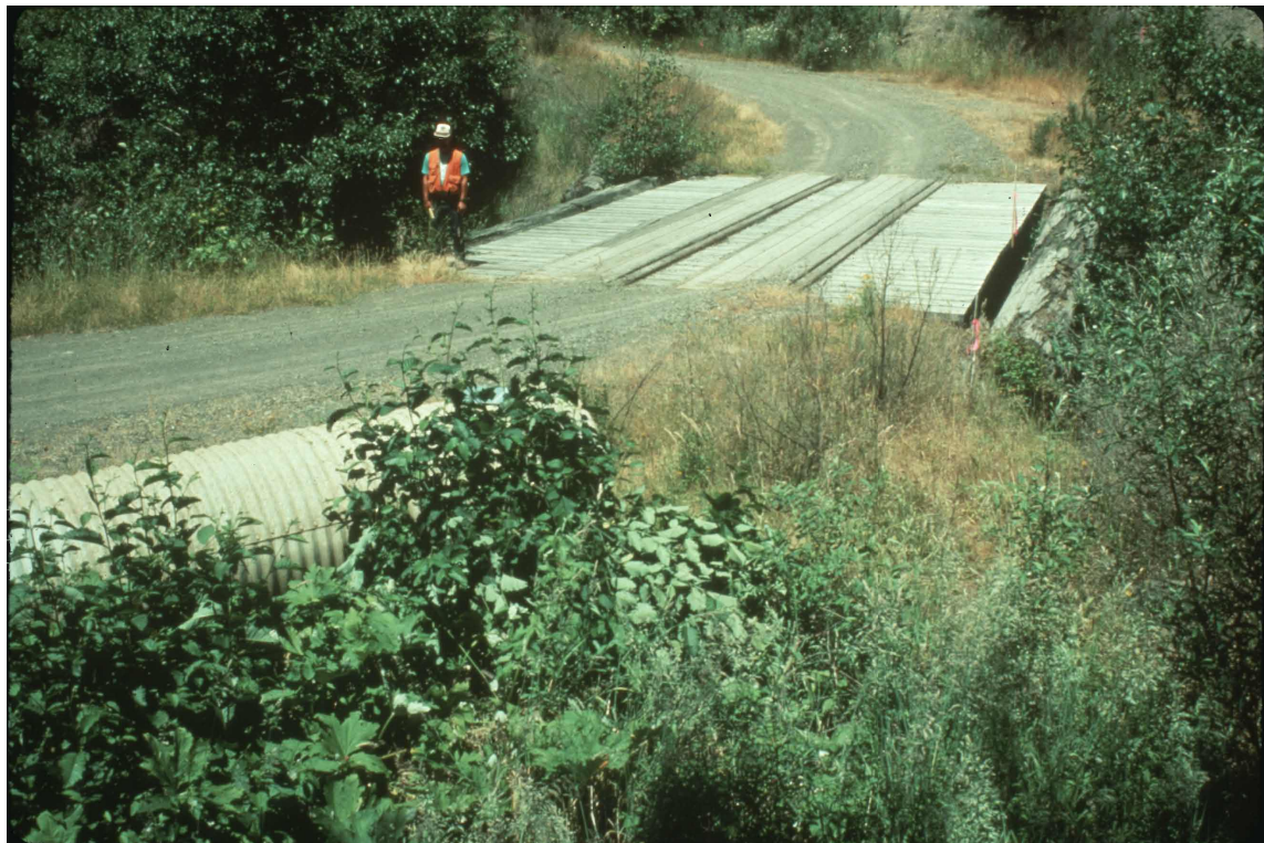
91-2 PP11b Pre H.E. 7/31/91 STA 157 + 00 Upsta -> CC Bridge 35mm DLS
