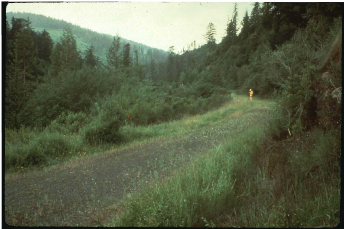
Unit: 88-2 PP8b Upsta Rd. STA 14+50 6-6-88 MH & RK 35mm
