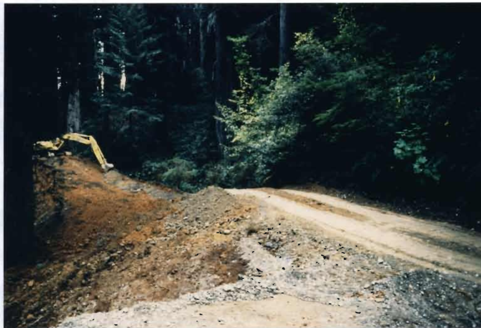
RX-8, Photo Point 45, 11/2/95. This photograph was taken during heavy equipment work. The large excavator is excavating fill from the upper end of the crossing and passing it to a bulldozer behind it that pushes the fill to a fillsite.
