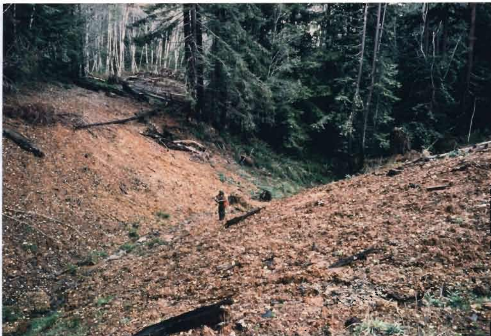
RX-7, Photo Point 35, 12/2/96. A large amount of wood, root wads, tires, and metal debris that had been pushed off the edge of the landing into the crossing has been removed and the edge of the landing pulled back to recreate the valley slope.
