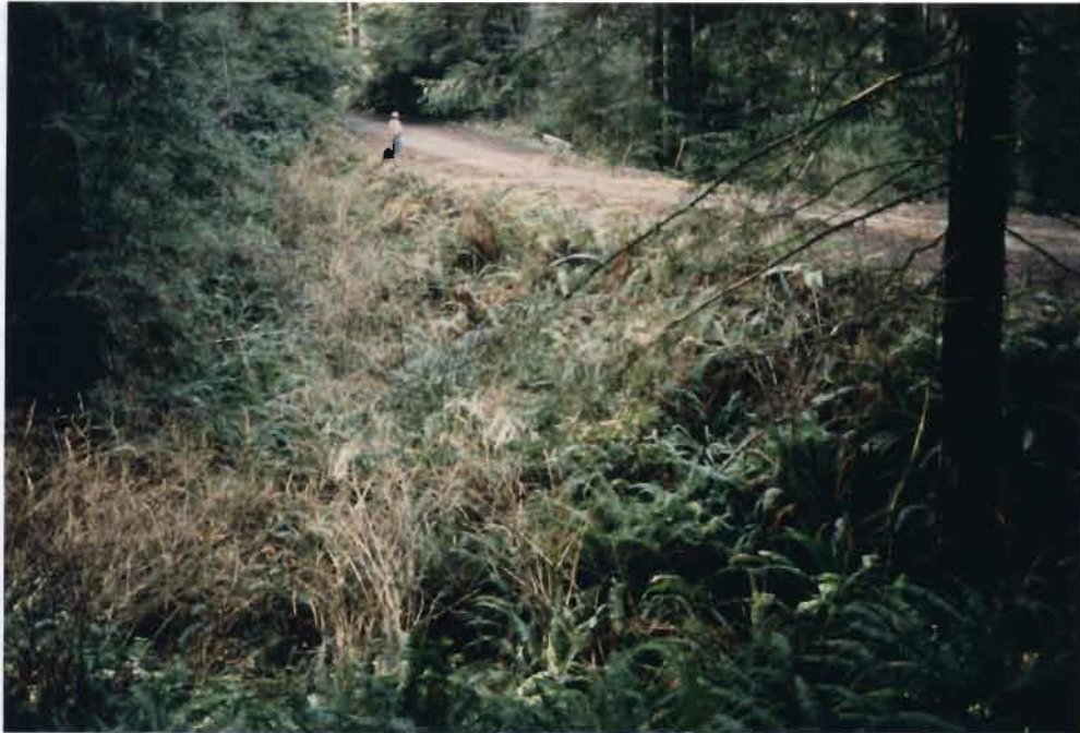
RX-8, Photo Point 43A, 3/1/94. This photograph is taken from the right bank of the crossing on the inboard side of the road fill.
