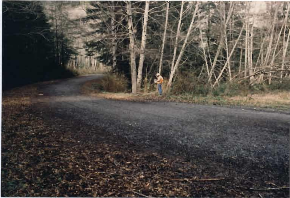
RX-7, Photo Point 35, 3/1/94. This crossing is at the left edge of the large landing on Ah Pah Road.
