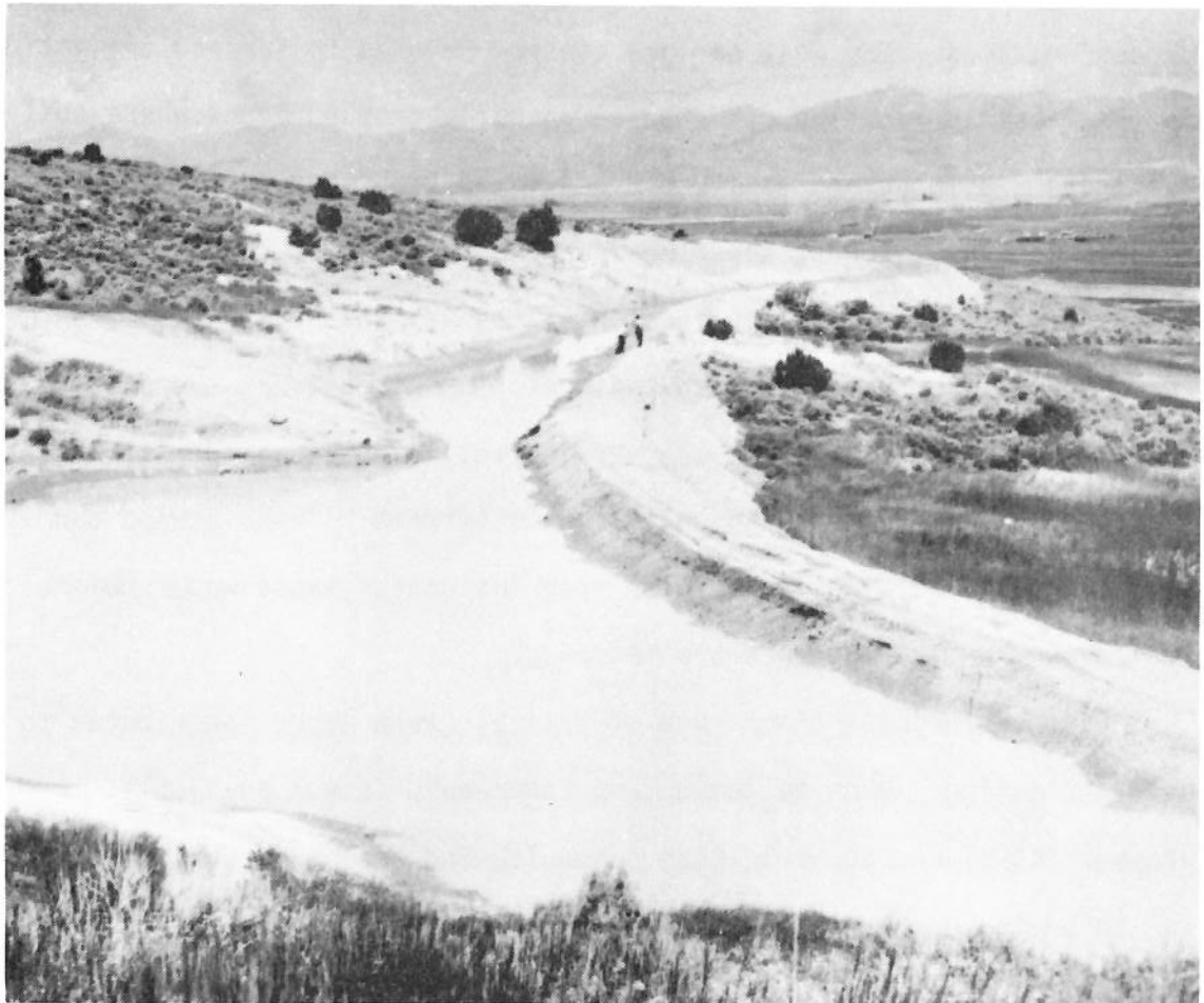
Diversion Terrace SCS Photo
