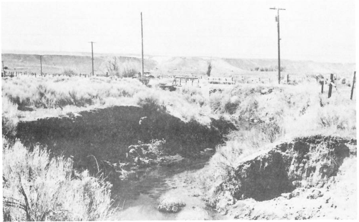
Channel Erosion SCS Photo
