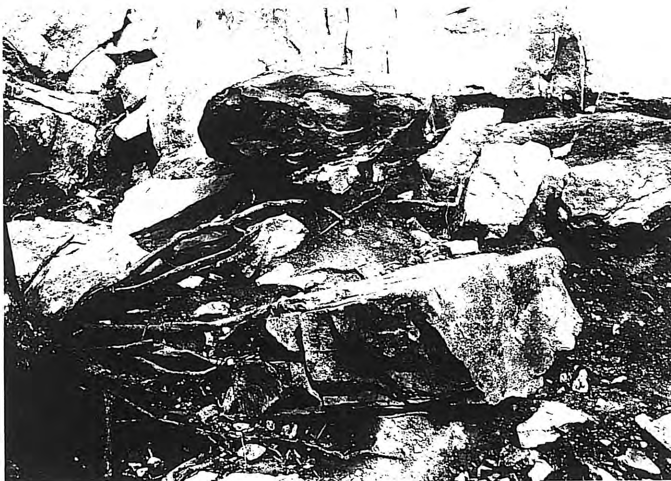
Figure 6. Soil Erosion at base of Sunset Rock.
