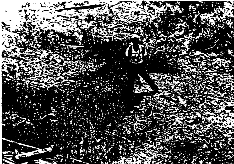
Figure 55: Grass seed and fertilizer were applied at equal rates on all areas of this skid road. The moist site on the left side of the photo has a fairly good grass cover developed; survival of grass is much poorer on the drier site on the right-hand side.
