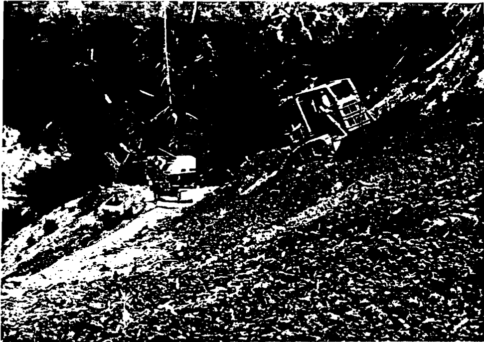
Figure 6: Excavated fill is piled along the inboard edge of the road and against the road cut bank. A tractor grades the fill to achieve a gentle outslope on the former road alignment.
