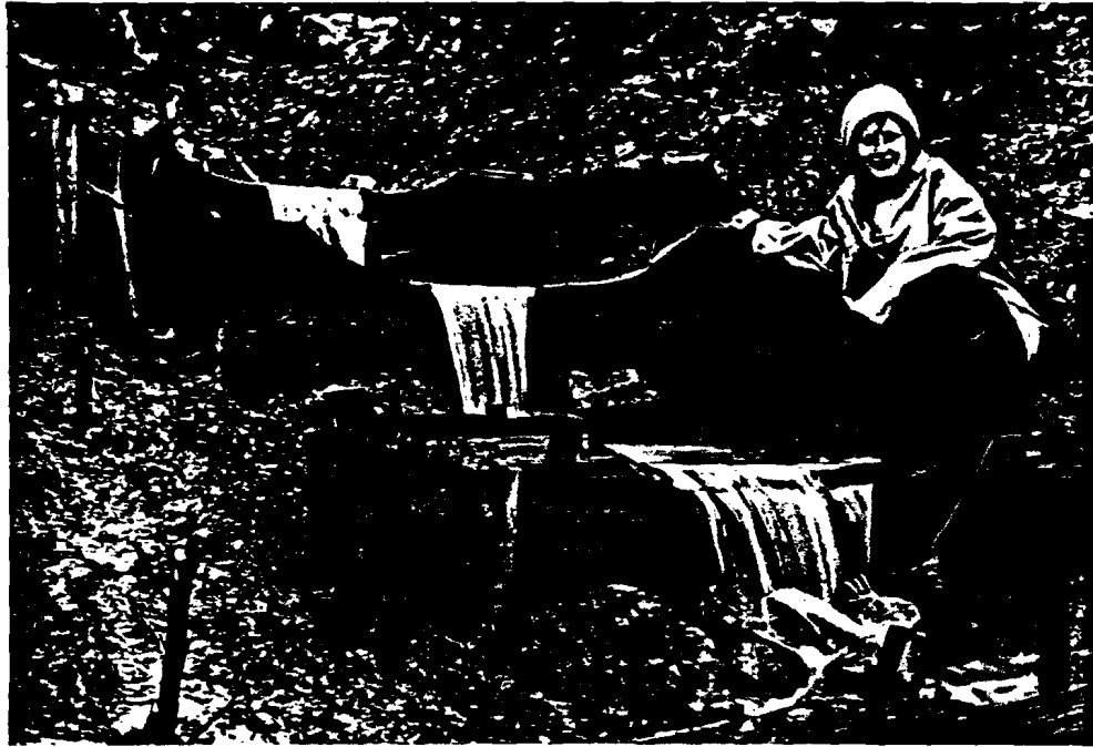
Figure 66: January, 1979 Miller Creek Unit check dams convey winter flows through broad, high-flow spillways. Large rocks are used as energy dissipators below spillways. Note willow stem cuttings on both channel banks.
