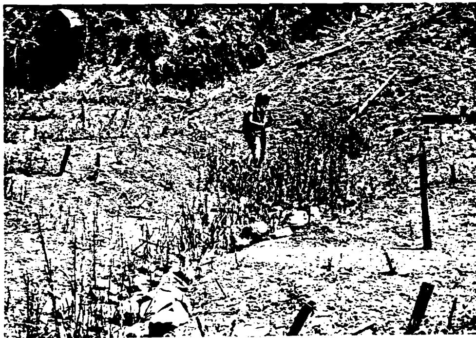
Figure 81: A thick stand of grass in a moist cross road drain adds support to the banks by its dense root mass. The grass and rocks trap fine soil particles that would otherwise be washed downstream.
