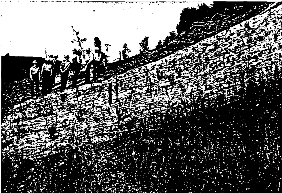
Figure 82: Redwood chip and brush mulch was spread on the outsloped road and Miller Creek, and was then covered with jute netting.
