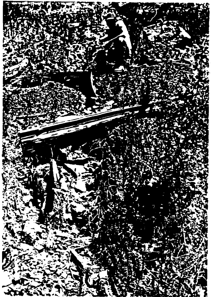
Figure 78: Emerald Creek Herringbone energy dissipator below cross road drain has been undercut. In this case, the distance between boards was too large, and the upstream sides of the slats were not protected by rocks.
