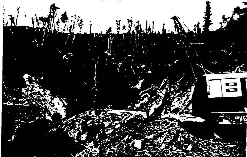
Figure 5: Because of its long reach, a dragline crane is used to lift unstable side cast road material and organic debris to the road bench.
