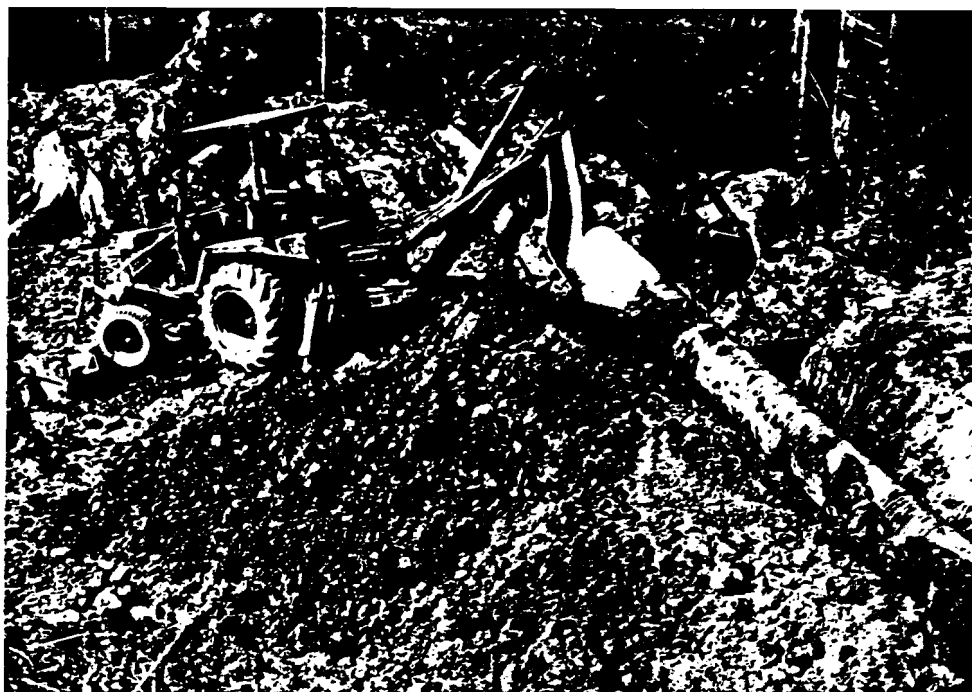
Figure 19: A backhoe excavated and removed culverts from the C-90 road, and smoothed out the resulting trough to form a cross road drain with gently sloping banks.
