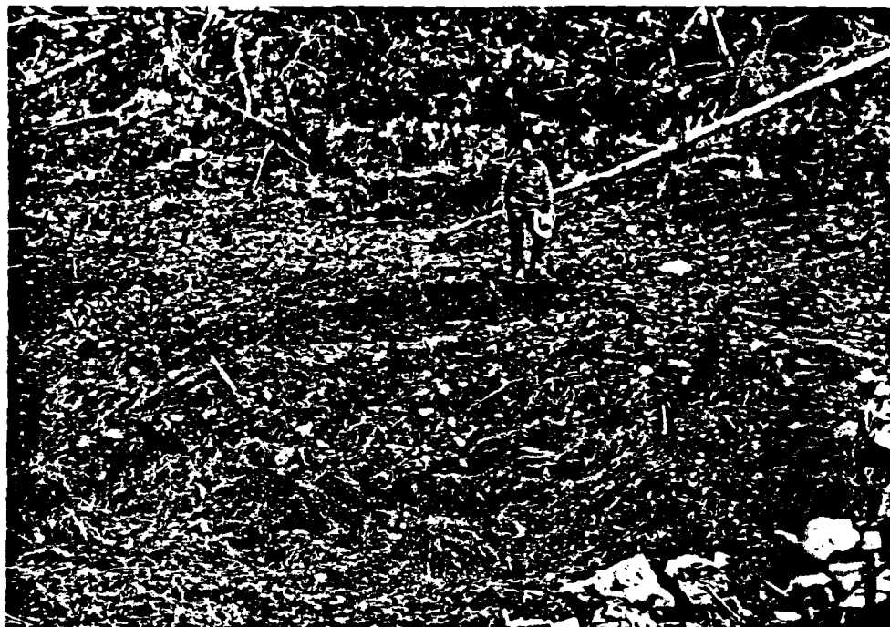
Figure 31: April, 1979. A small slump occurred on a recently wattled slope in an area with few cross road drains.
