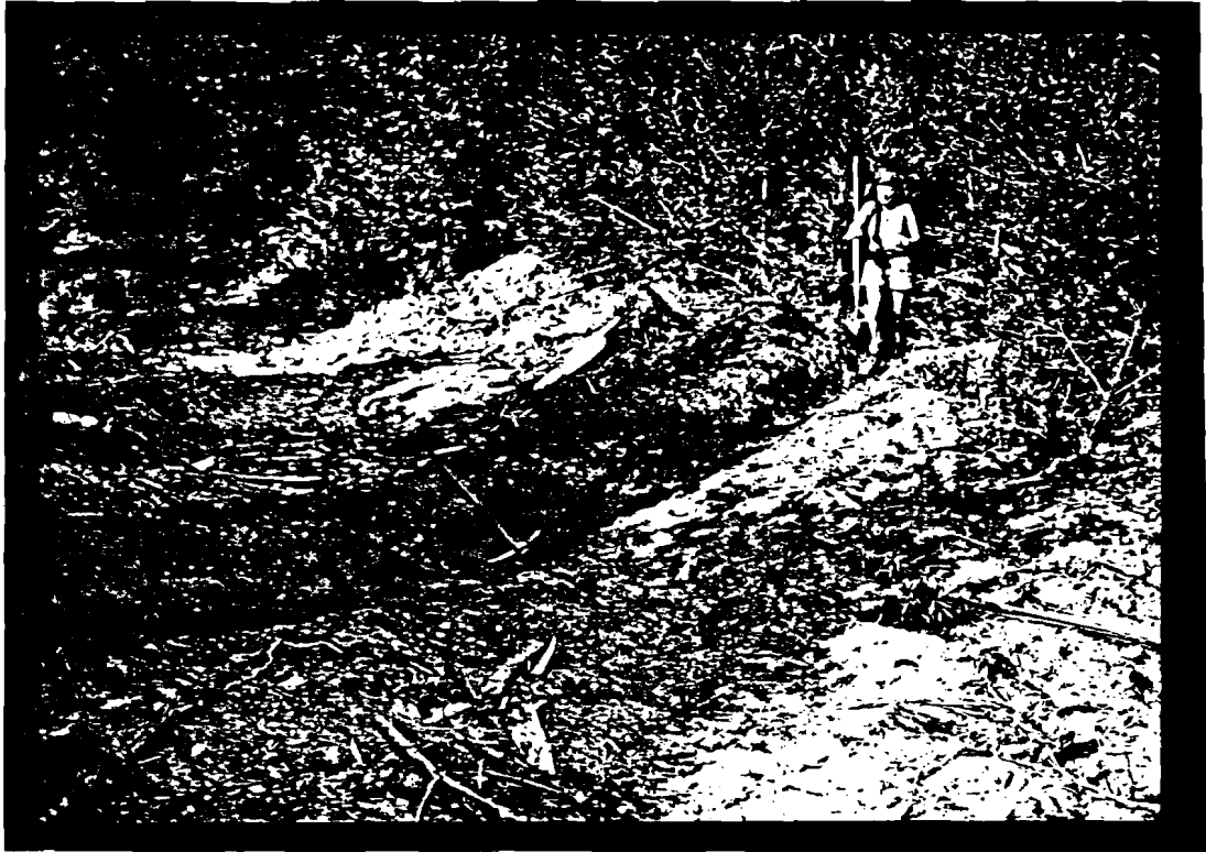
Figure 61: June, 1979 A hand-constructed waterbar on the Lower Bond Creek Unit. Runoff from the skid road is diverted into heavily vegetated area behind the person in the photo.
