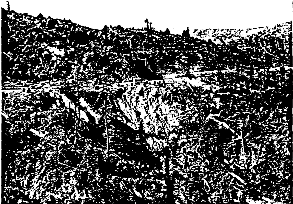
Figure 56: PP3 10/2/78 View towards C-Line landing prior to any rehabilitation work. Part of the landing failed, leaving much of the organic and inorganic debris perched precariously.
