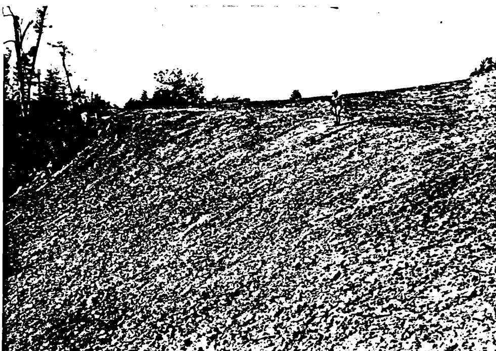
Figure 13: PP3 3/12/79 After photograph of log landing. Edge of landing has been pulled back and fill material was outsloped. Drainage of runoff from the landing has been improved. Willow wattles were planted on the steep slopes below the former landing.
