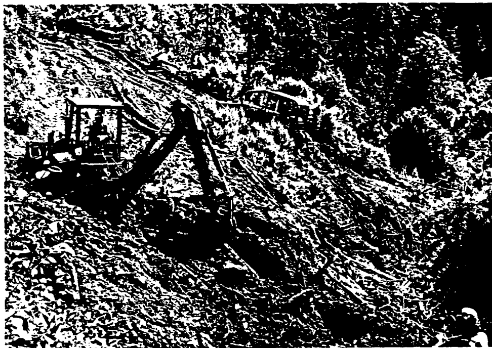
Figure 38: A small backhoe is used to excavate road fill and organic debris from stream crossings. Stream banks are recontoured to achieve stable slopes. The cat in the background of the picture is winching large debris from the channel before the backhoe does the 'finish-up' work in clearing the channel.
