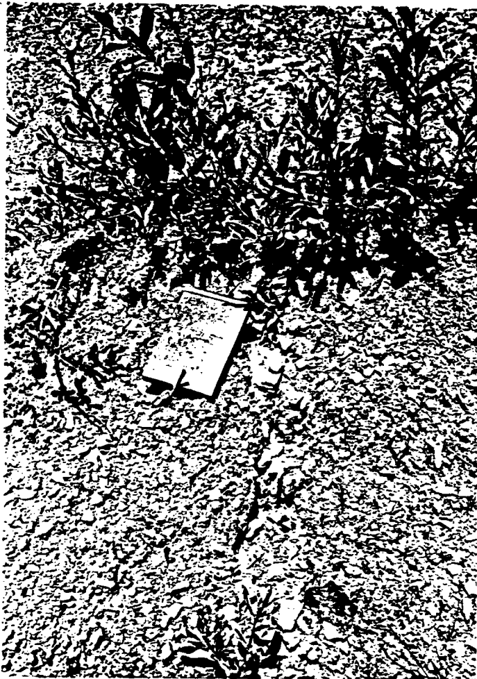
Figure 35: Although willow wattles can disperse small amounts of runoff and impede rilling, they are less effective when subjected to concentrated runoff. Here, a rill beginning upslope of a wattle row carries enough runoff to undercut the wattle and continue rilling downslope.
