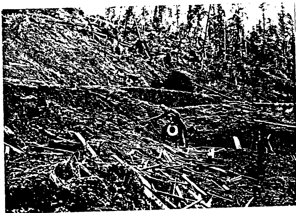
Figure 32: April, 1979. The outside edge of a landing failed where instability had previously been seen (see Figure 30 for comparison). The man's hand points to a cross road drain that has been truncated by the scarp of this failure.
