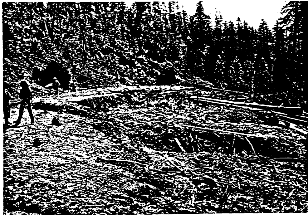
Figure 30: PP14d 3/19/79 After rehabilitation, culvert has been removed and cross road drains have been constructed to drain surface runoff from the site of the failure. In addition, a drainage ditch was dug at the toe of the cut banks to direct runoff into cross road drains. The deep-seated failure was not addressed except through upslope drainage diversions.
