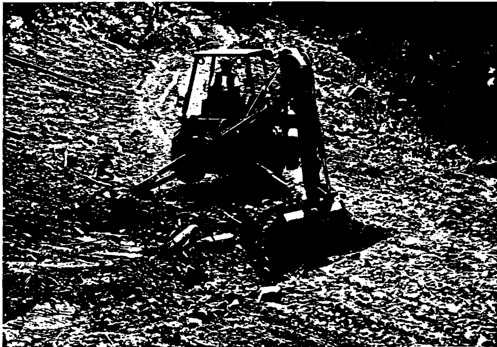
Figure 20: To prevent runoff from concentrating in the inboard ditch, cross road drains are excavated along the C-90 road by a backhoe.
