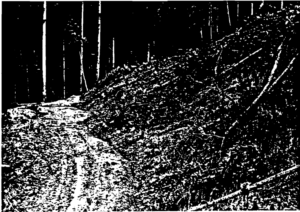
Figure 21: PP16a 8/23/78 C-90 road prior to rehabilitation is showing signs of instability. Small cut bank failures are blocking the inboard ditch. Note the scarp of a road fill failure behind the person at the left of the photo.
