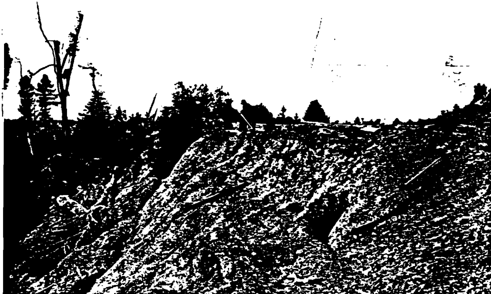
Figure 12: PP3 8/22/78 Before photograph of oversteepened edge of log landing. Some fill material and organic debris have already failed downslope. In addition, water continued to pond on the landing, and tensional cracks suggested future failure of the hillslope.
