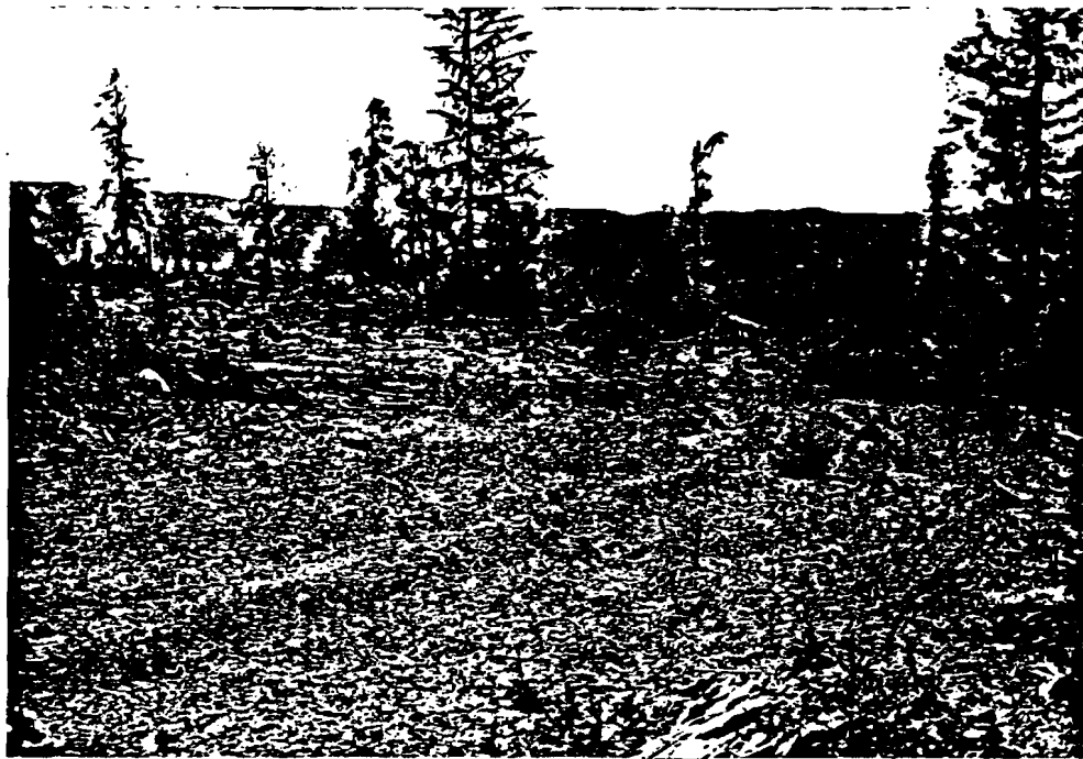
Figure 16: PP22b 8/22/78 Before and after sequence of a rocked haul road that was disaggregated (ripped) by a D-8 cat tractor to promote revegetation and infiltration of runoff. Note the paucity of vegetation on the compacted road surface even following 5 to 7 years of non-use.
