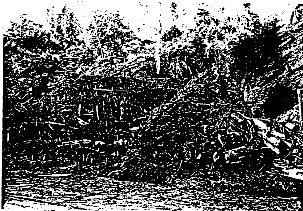
Figure 44: 1/4/79 Note check dams in channel, willow wattles on slope, and staggered planter boxes staked into slope.
