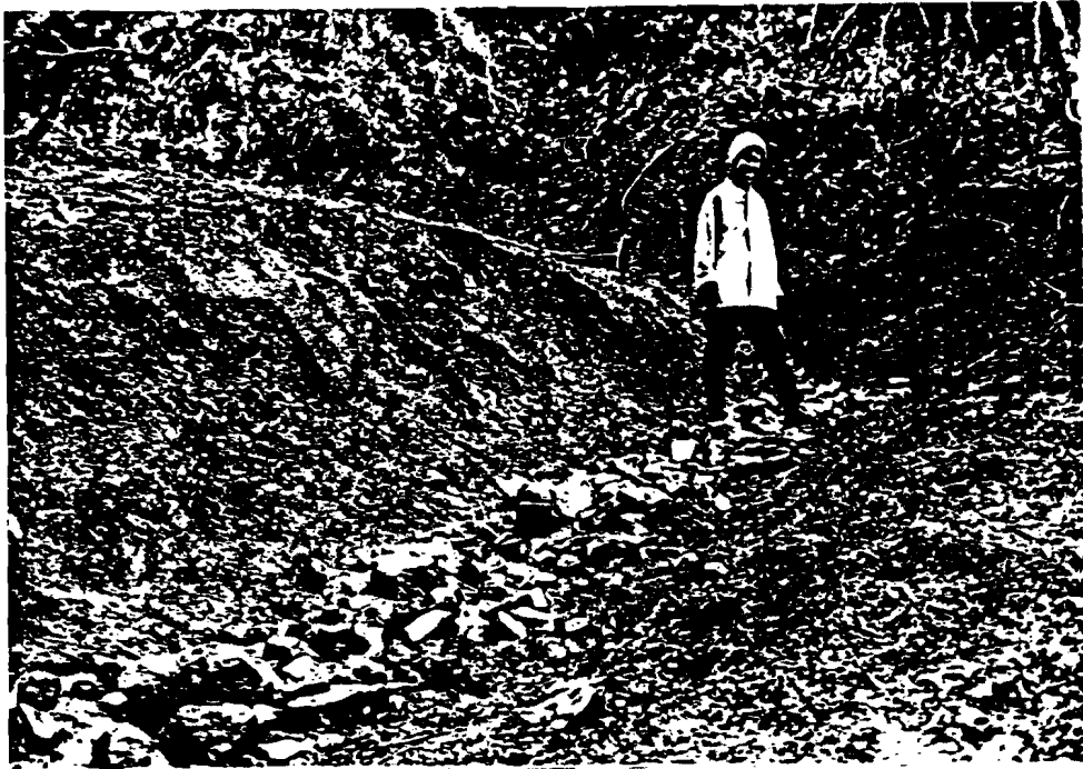
Figure 80: Manually-placed coarse rock on the bed of a cross road drain prevents downcutting of the channel bed while allowing unhindered flow of runoff through the drain.
