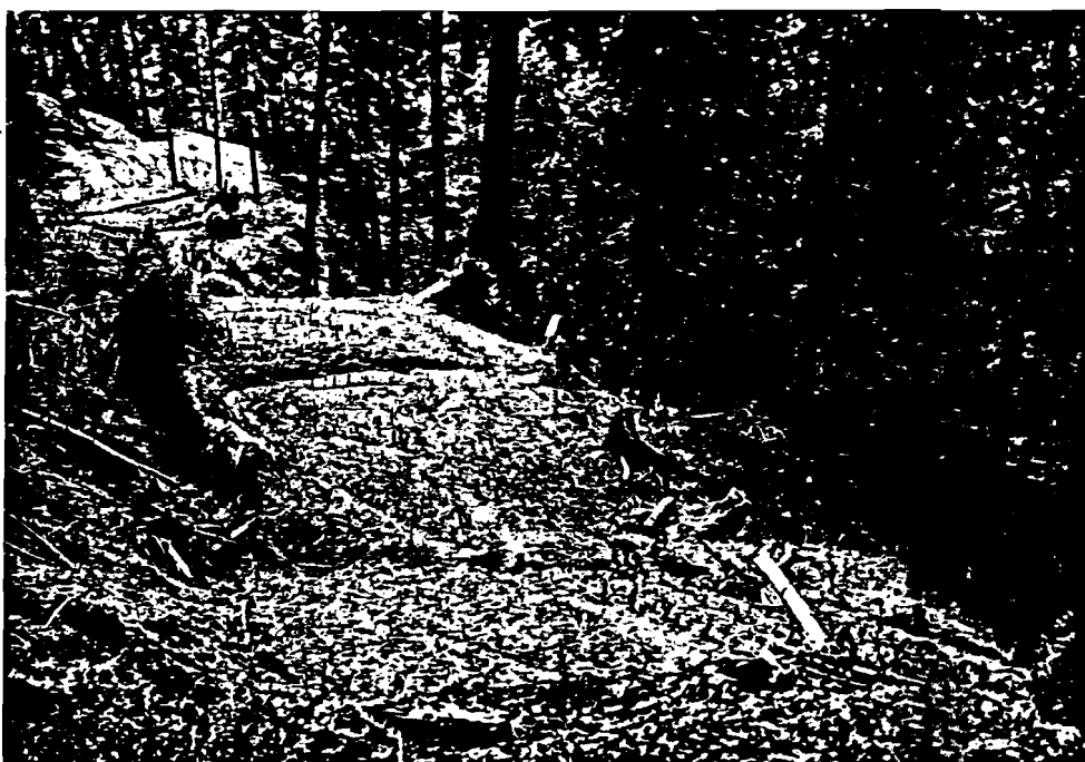
Figure 26: PP16c 3/19/79 After rehabilitation, C-90 road has been decompacted and outsloped, and the inboard ditch has been filled in. Surface runoff now crosses the removed road through cross road drains rather than concentrating and flowing along road alignment.
