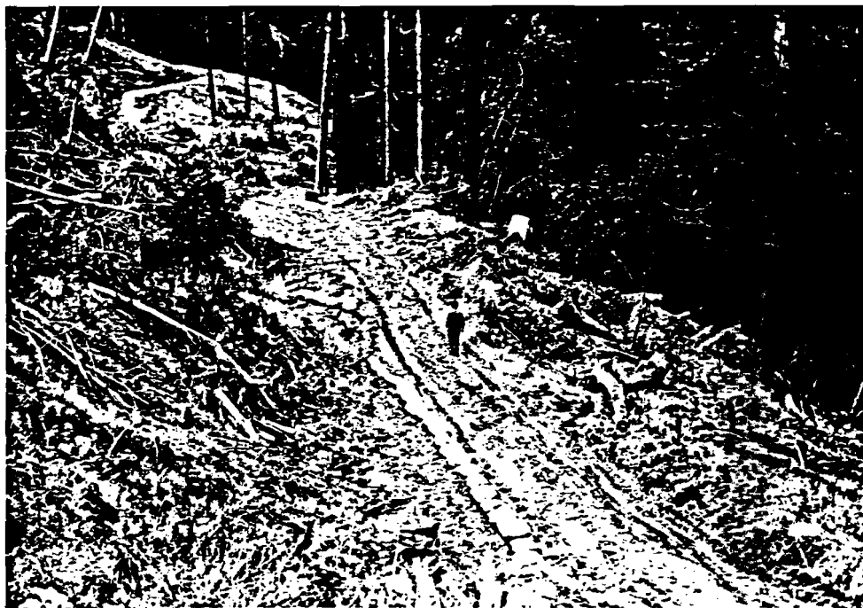
Figure 25: PP16c 8/23/78 C-90 road prior to rehabilitation. Sandbags line the unstable inboard ditch of the rocky haul road.
