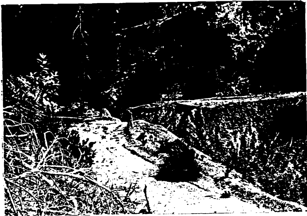
Figure 8: PP5a 8/22/78 Before photograph of former culvert in Drainage 6. Culvert became plugged with debris and winter flows washed out about 800 cubic yards of road fill into the stream channel.
