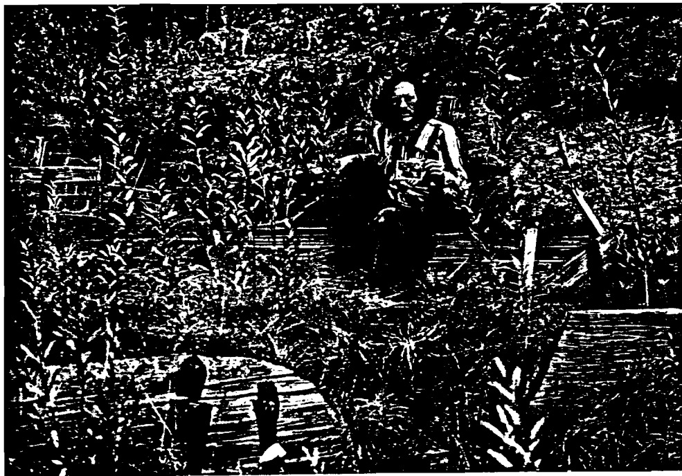
Figure 68: September, 1979 Same series of check dams as figure 66 showing revegetation after one season. Willow ( salix , spp.) have sprouted from stem cuttings while horsetail ( Equisetum , spp.) invaded naturally.
