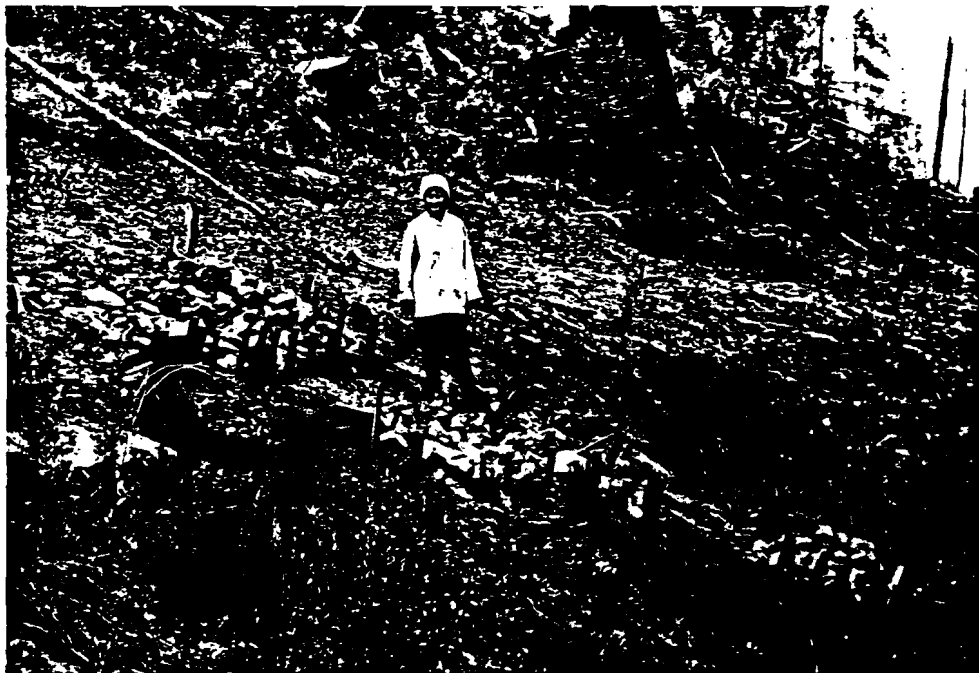
Figure 79: Emerald Creek CRD 15 Piles of rock anchored to the slope below a cross road drain, filter runoff through them and dissipate erosive energy.
