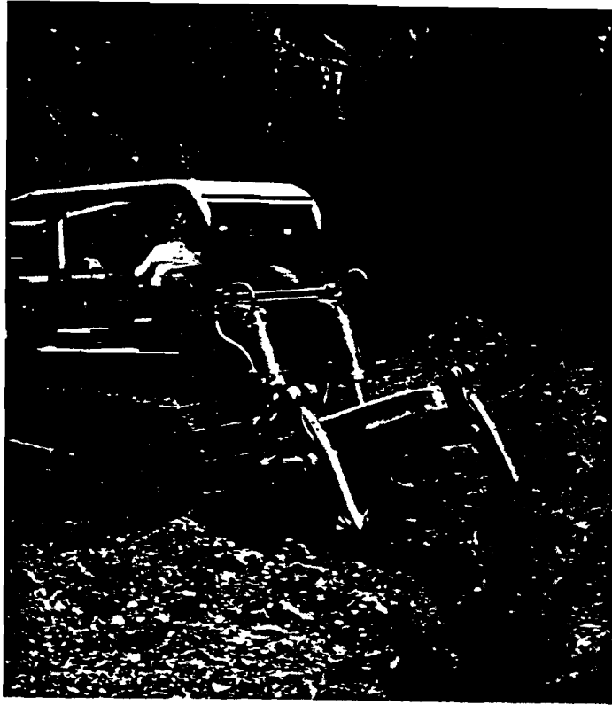
Figure 4: Most logging roads are surfaced with eight to twelve inches of rock and must be disaggregated to promote infiltration and revegetation. Here, a D-8 Cat decompacts the C-10 road with its ripper teeth.
