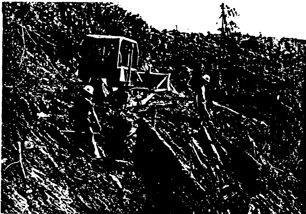
Figure 37: Organic debris that was incorporated in road fill is winched out of stream crossings by a caterpillar tractor.
