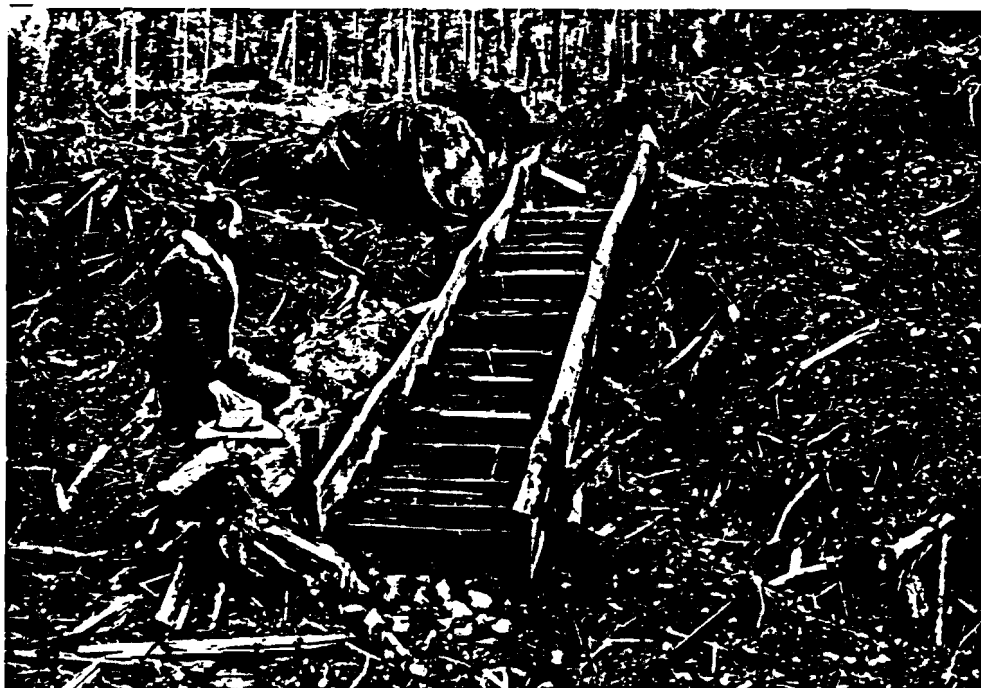
Figure 72: Type 4 Water Ladder
