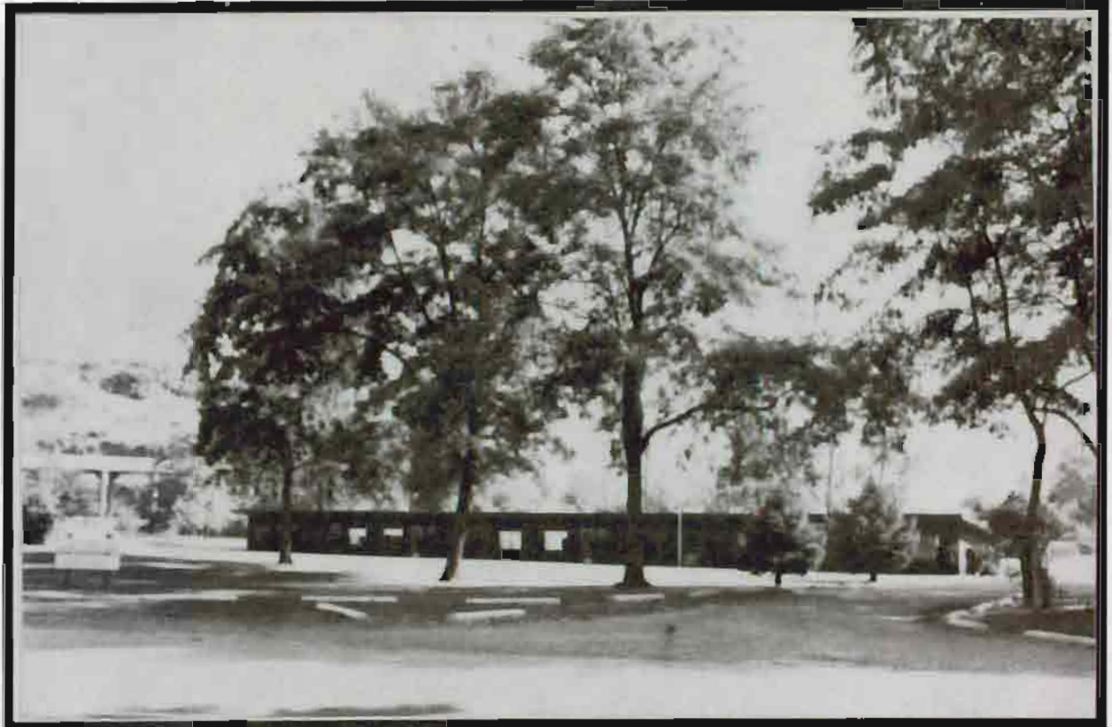
Park administration building . . .
