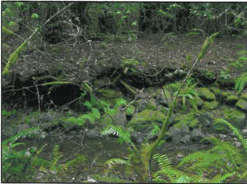
Figure 16. Downstream end of riprap section R9. Note the rock slumping into the channel and the bank scour on the left.
