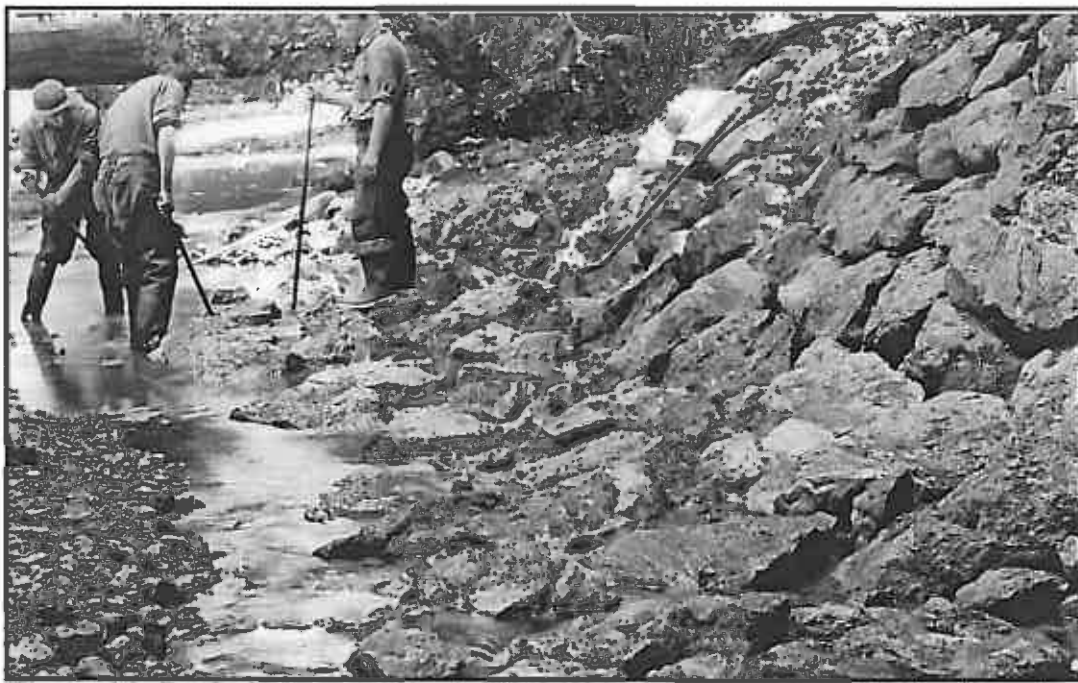
Figure 14. Rock riprap armoring the stream bank and extending into the channel as depicted in Figure 13 (from NPS Archives).
