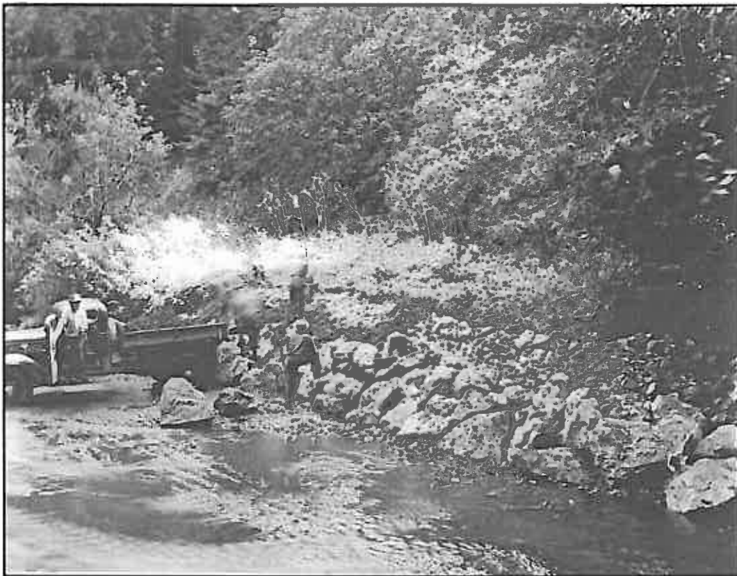
Figure 10. Equipment working in streambed during CCC riprap construction ca. 1937, note the bed and bank disturbance (from NPS Archives).
