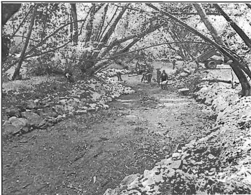
Figure 9. CCC workers installing rock riprap along the banks of Redwood Creek. Note the lack of bank vegetation and the truck on the bank, showing bank disturbance, also the machinery in the creek. ca. 1934 (from NPS Archives).
