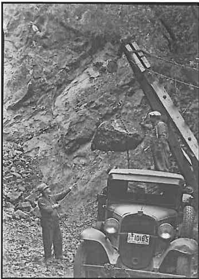
Figure 7. CCC workers loading rocks at the Kent quarry for riprap in Muir Woods ca. 1934 (from NPS Archives).
