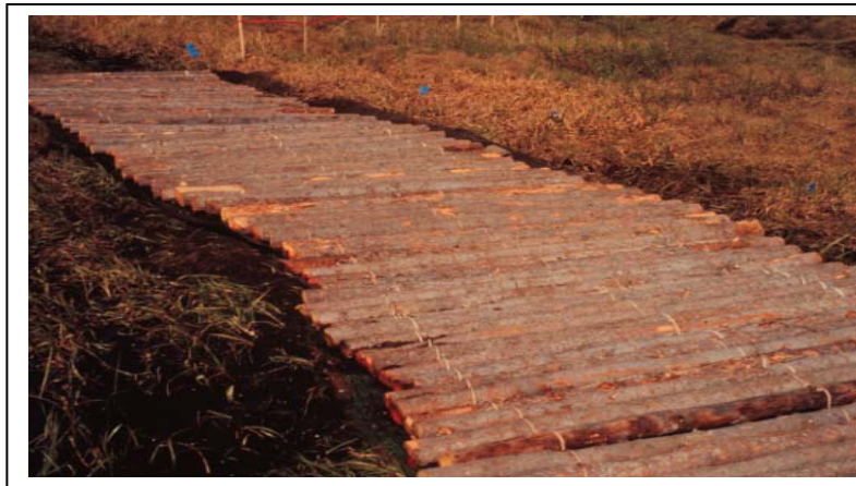
Figure B. Woven Corduroy tested for ATV trail mitigation in Wrangell-St. Elias National Park and Preserve.
