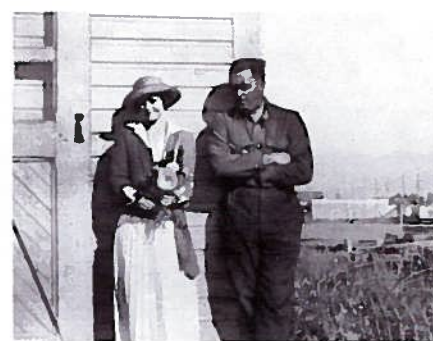
National Park Service photograph
