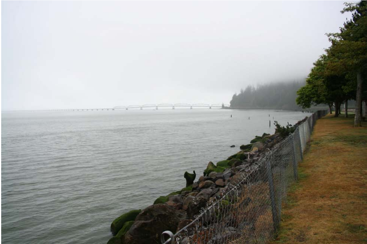
Figure 66. Rock revetment at Dismal Nitch.
