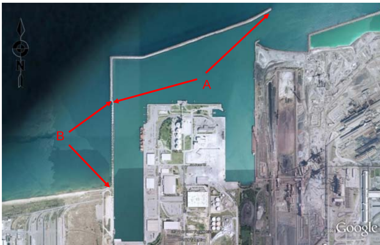
Figure 54. Port of Indiana-Burns International Harbor.
