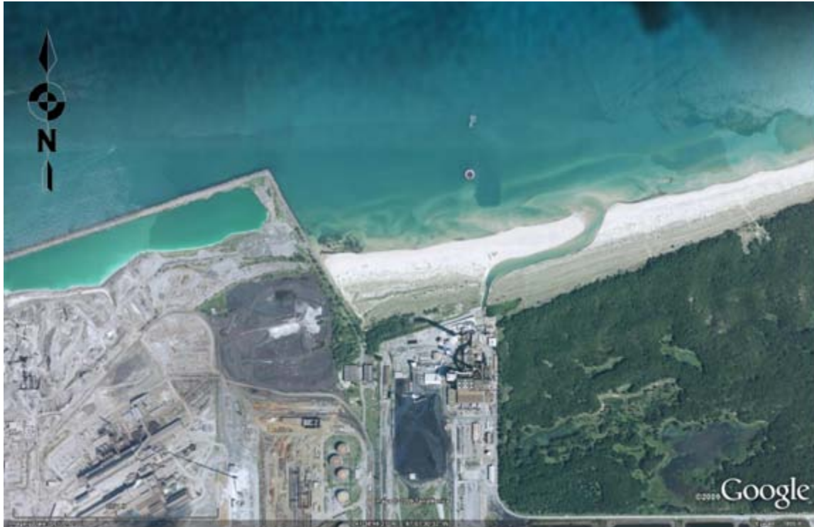
Figure 59. Bailly Generating Station water intake structure.
