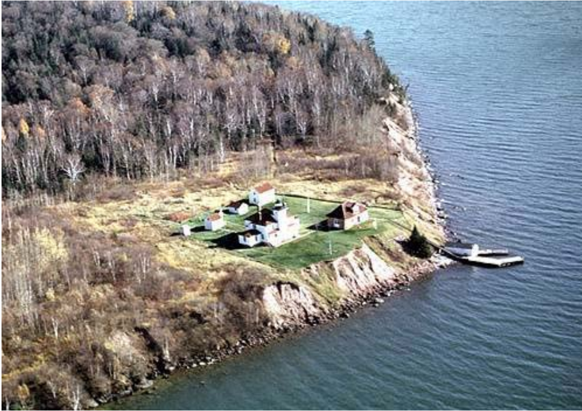
Figure 3. Raspberry Island Lighthouse before construction.
