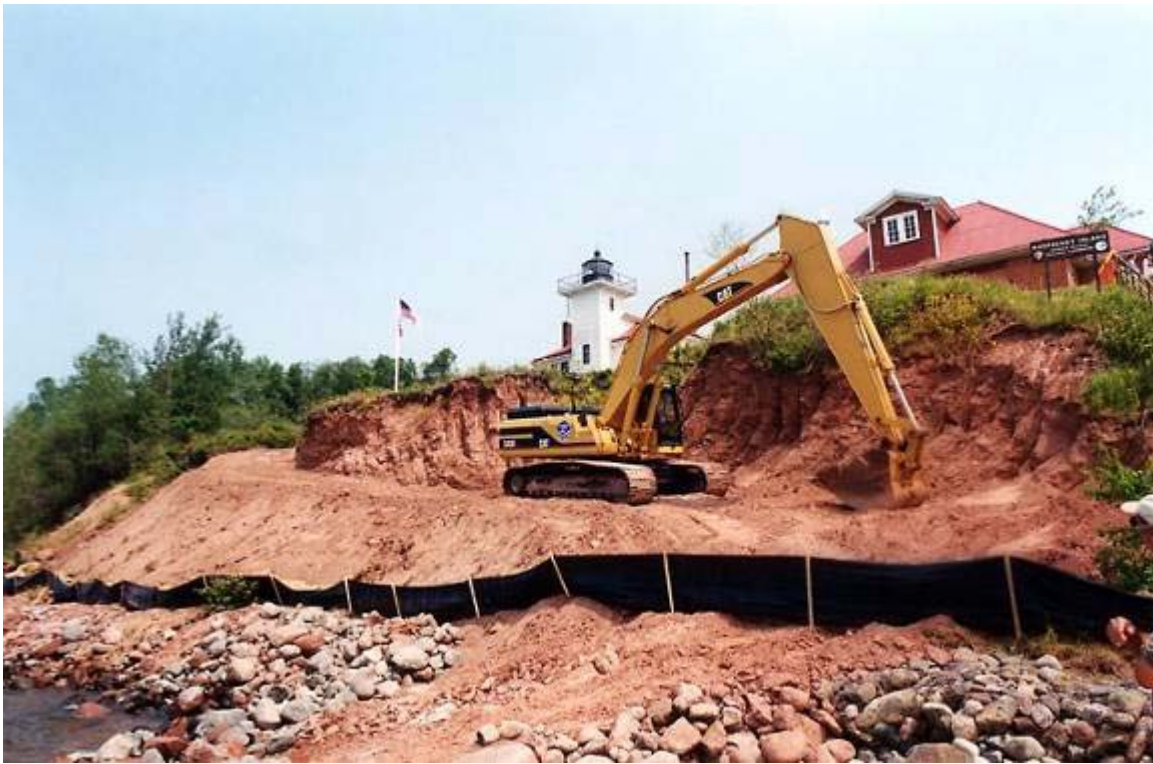
Figure 4. Raspberry Island Bank Stabilization Project.
