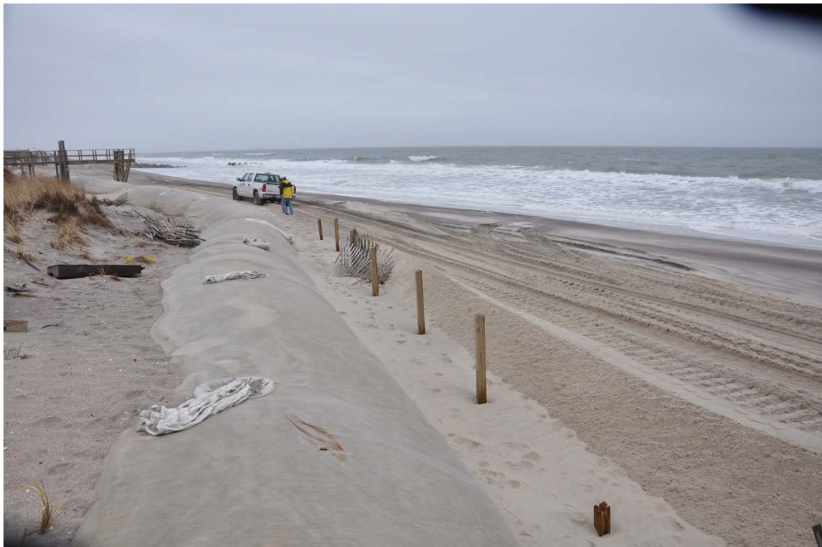
Figure 37. Geotextile structure at Ocean Beach.
