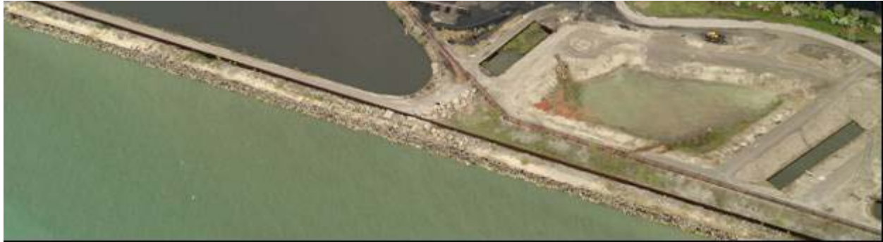
Figure 49. Rock revetment west of Michigan City Harbor.
