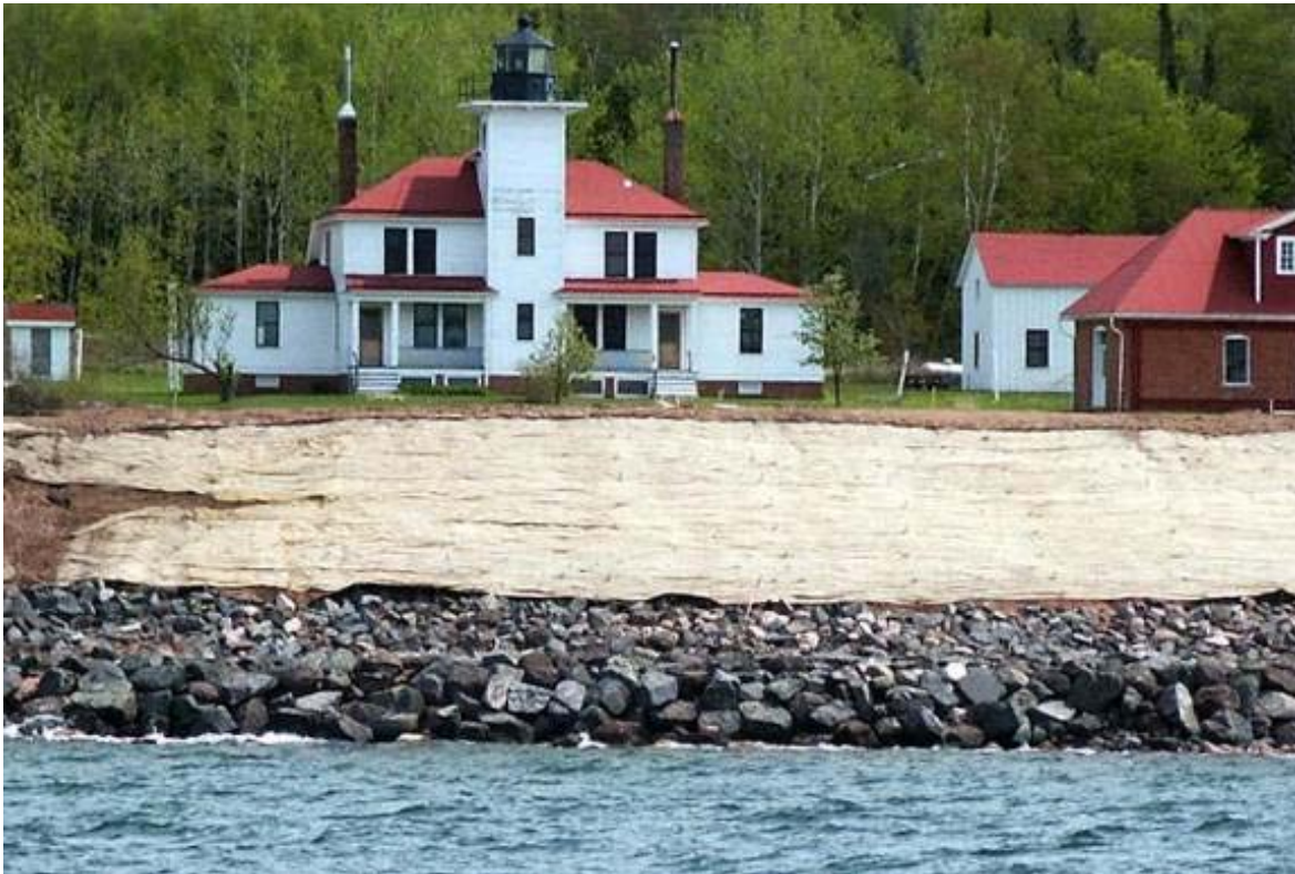
Figure 5. Raspberry Island Bank Stabilization Project during construction.
