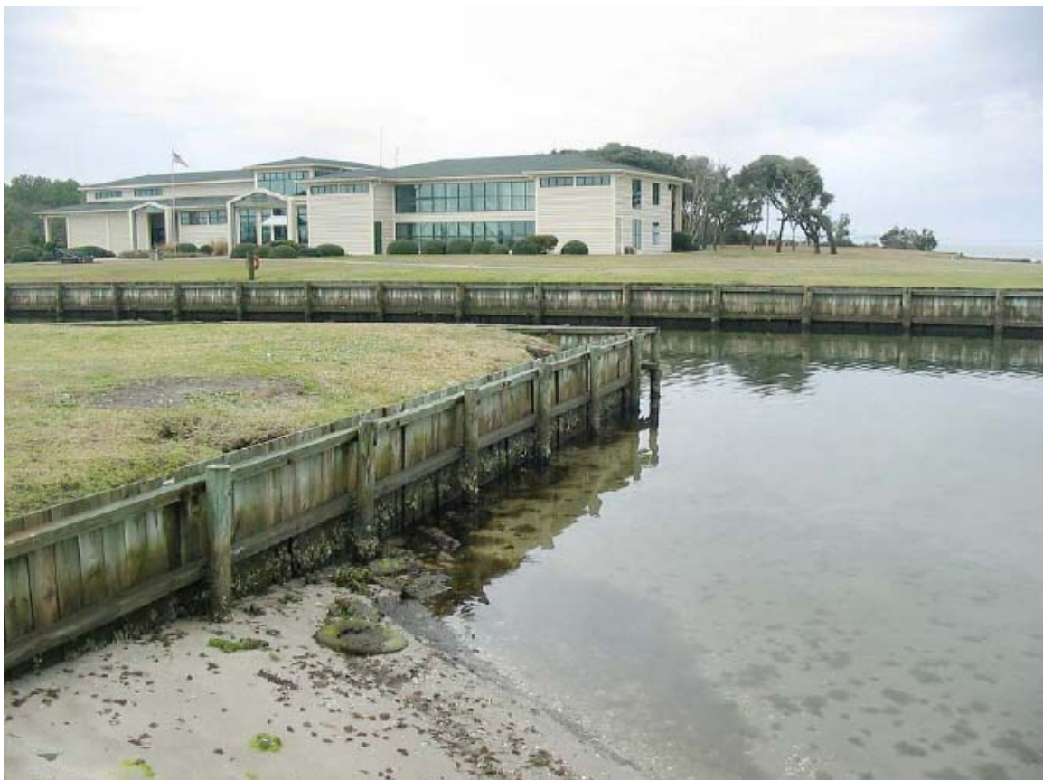
Figure 19. Cape Lookout National Seashore Park Headquarters
