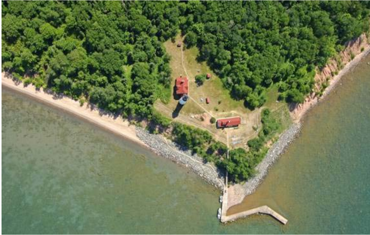
Figure 7. Outer Island Bank Stabilization.
