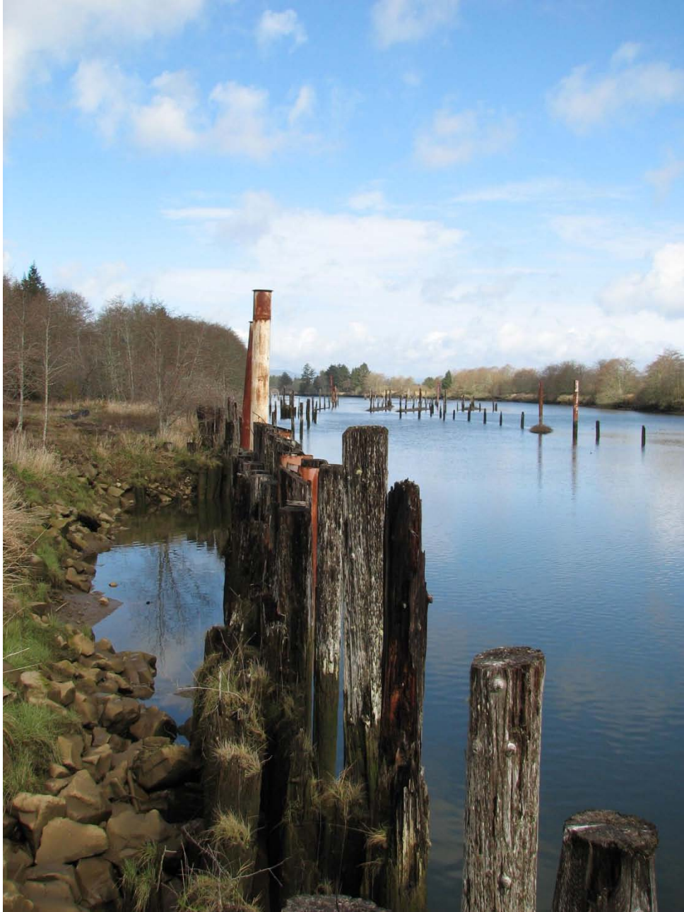
Figure 68. Pilings and Rip Rap Revetment at Netul Landing.
