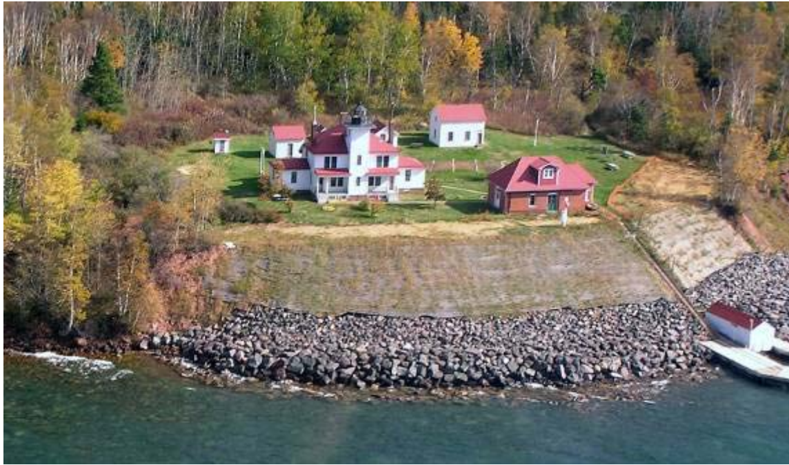
Figure 6. Completed Raspberry Island Bank Stabilization Project.
