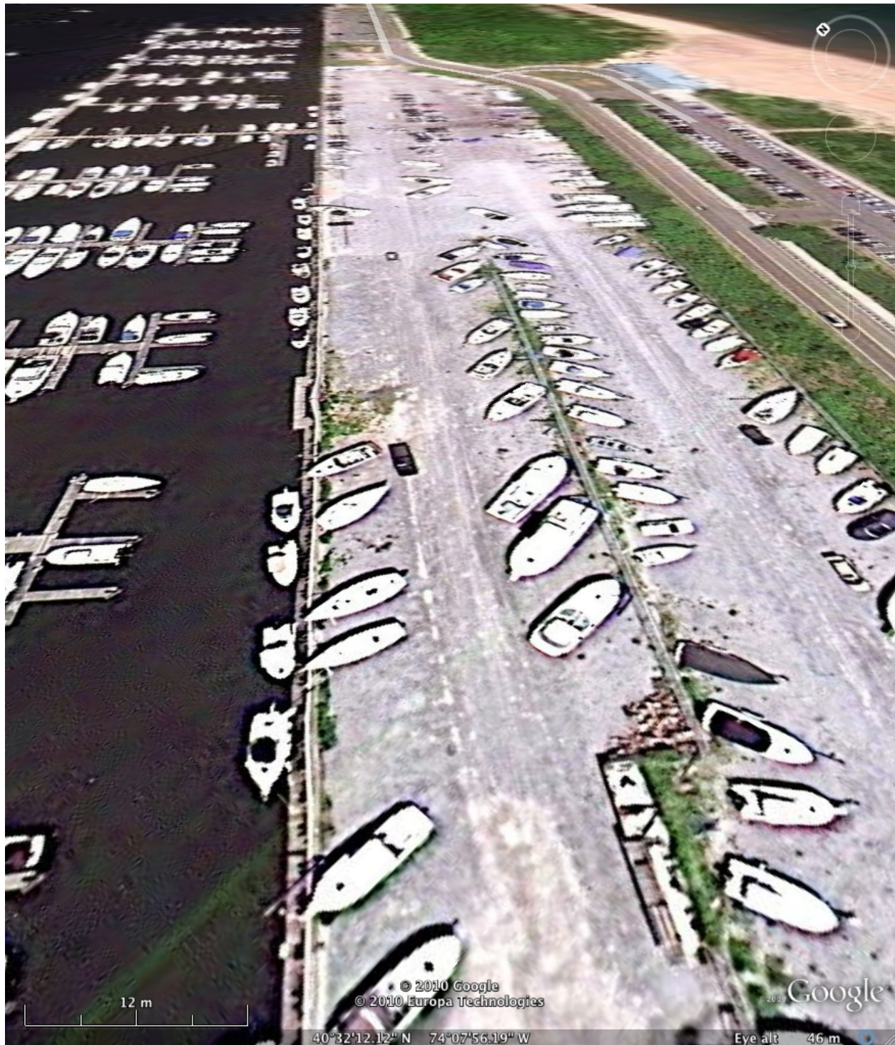
Figure 6. The shifts of the bulkhead and its pilings toward the marina basin are evident in the foreground of this photo and in the middle ground. Date of photo is unknown.
