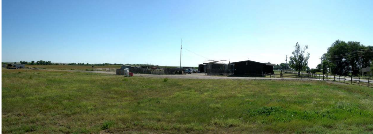
Figure 26. View of the park employee entrance gate as it passes along the maintenance and administration buildings. The flooding ditch is parallel to the road and between the road and buildings.
