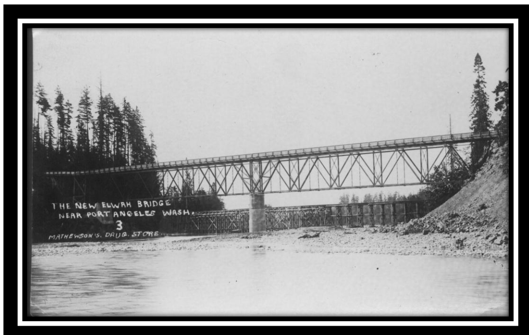
Figure 34 One-lane bridge with railroad bridge behind it, circa 1914 (OLYM-POL.013.001)
