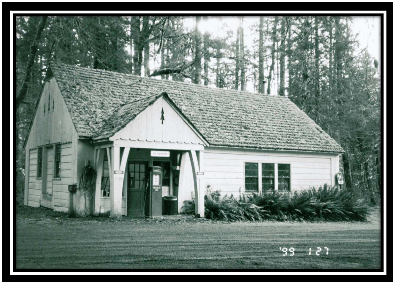
Figure 65 Elwha Ranger Station Historic District Oil, Storage, and Service building (OLYM18381015)
