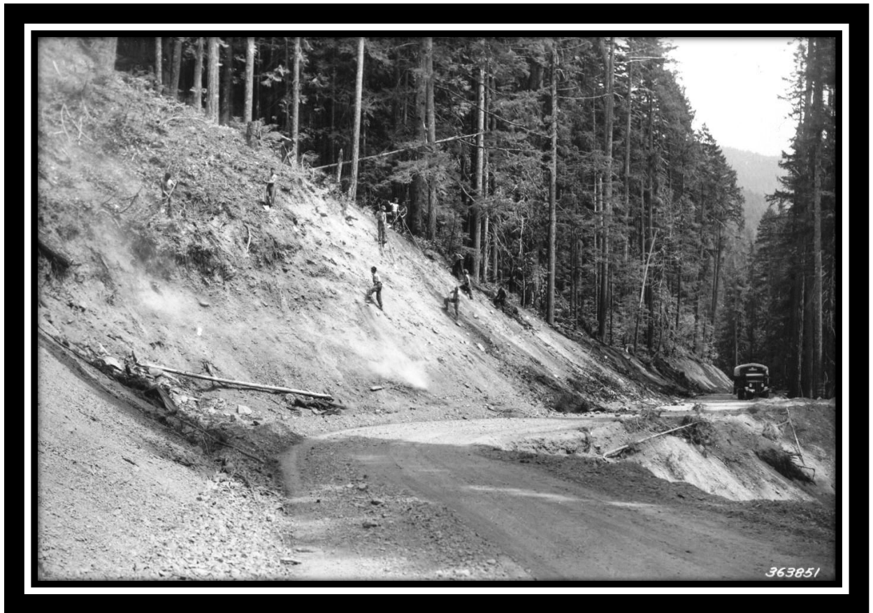
Figure 56 CCC working on Hot Springs Road (OLYM-FOR.SER.105)
