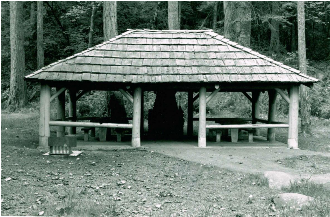
Figure 64 Altair Community Kitchen (OLYM18381078)
