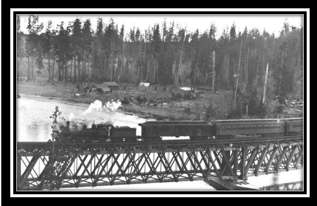
Figure 36 Railroad Bridge across Elwha River
