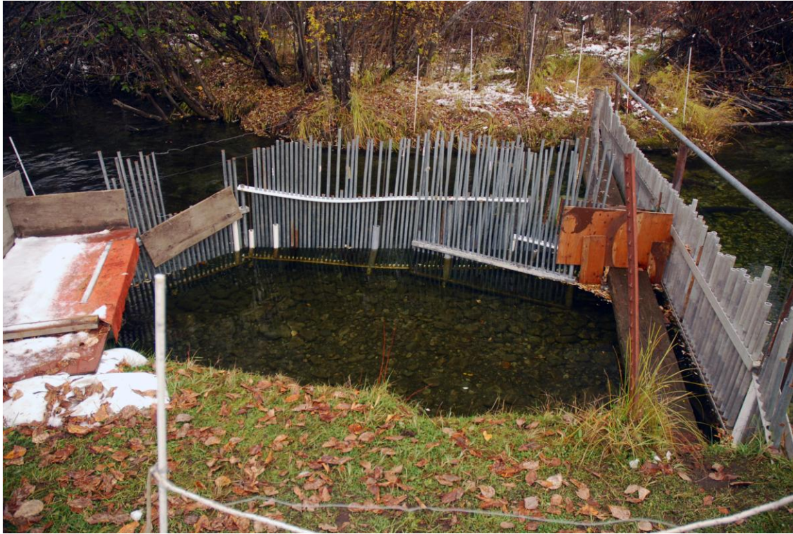
Figure A 3. Overview of the sampling box that is attached to the weir. Fish are allowed into the sampling box by removing appropriately located pickets in the weir. Note the work area to the left, where sampling occurs after fish are captured. After sampling, fish are returned directly to the water upstream of the weir structure.
