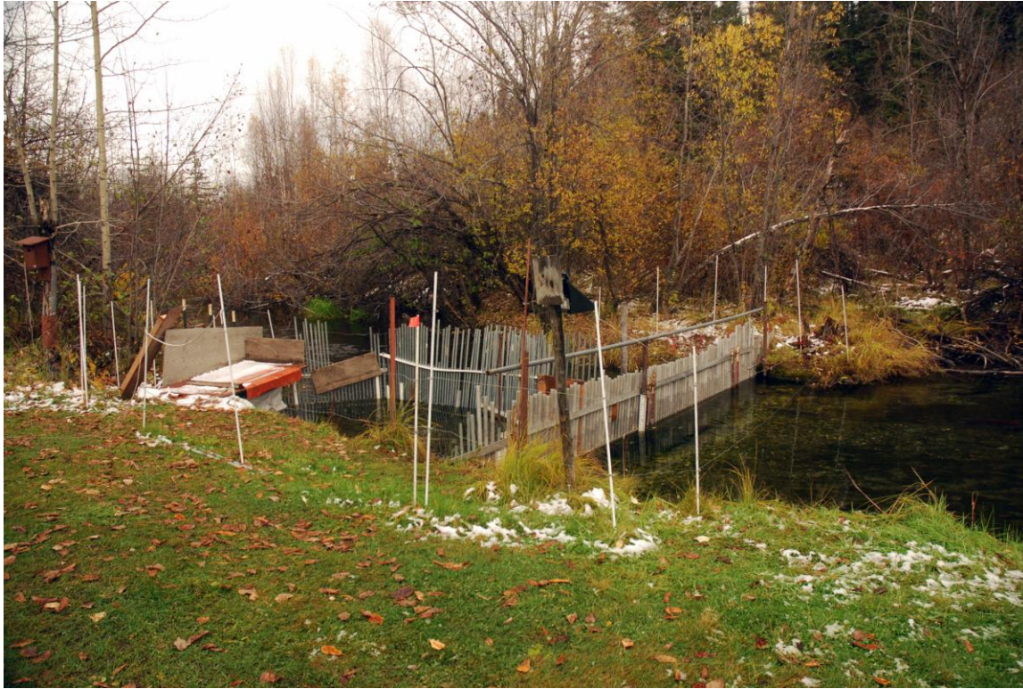
Figure A 2. Overview of the weir when operational. Stream flow is from left to right. Note placement of electric bear fence (strung on white poles). The bear fence completely surrounds the weir. The weir itself stretches straight across the stream. Additional framing and pickets are used to construct the sampling area seen on the left.
