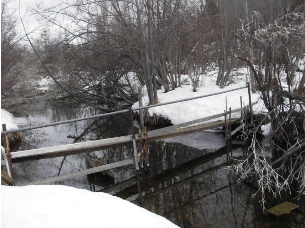
Figure A 1. View of weir framework during winter.
