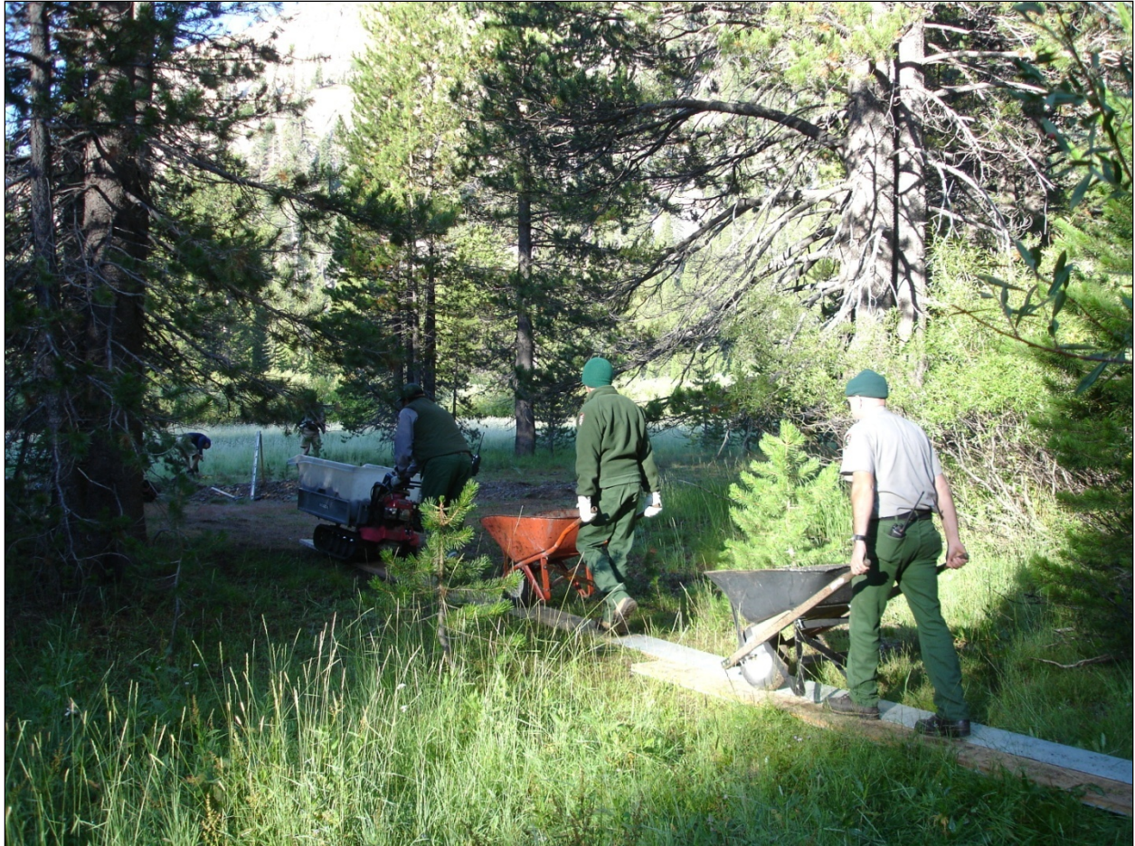
Figure C-2. DEPO staff carting concrete for the footing of the Soda Springs weather station, Devils Postpile NM. Note the travel boards used to reduce impact to the surrounding area. 17 August 2005
