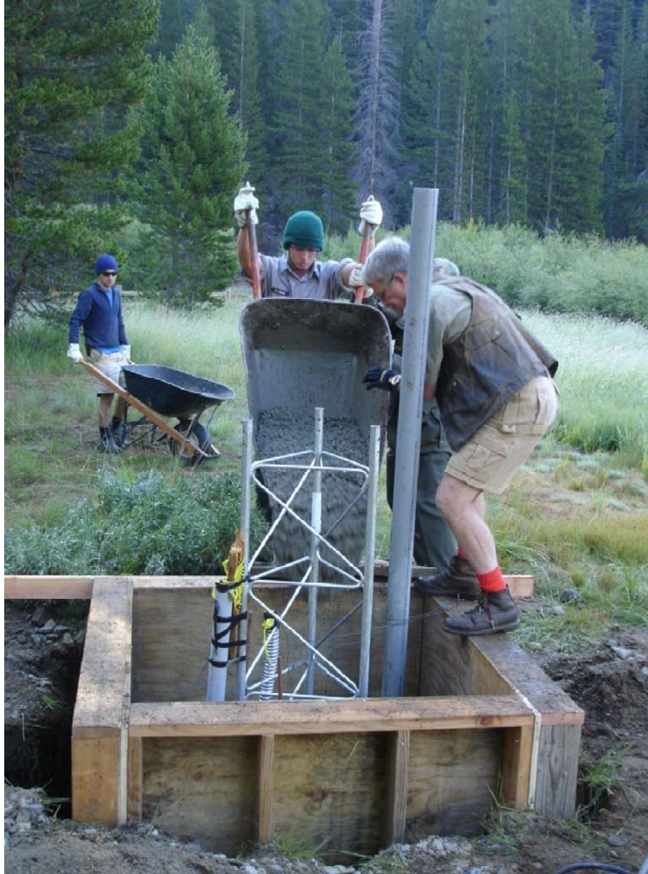
Figure C-3. DEPO maintenance worker Colin Leslie pours one of the dozens of loads of concrete needed to create the footing for the Soda Springs weather station, Devils Postpile NM. 17 August 2005
