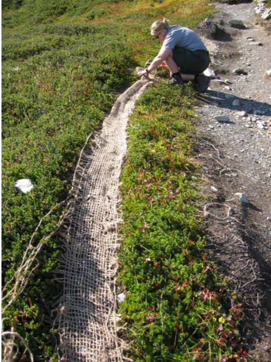
Jute Mesh Installed Along a Parallel Trail. NPS Photo.
