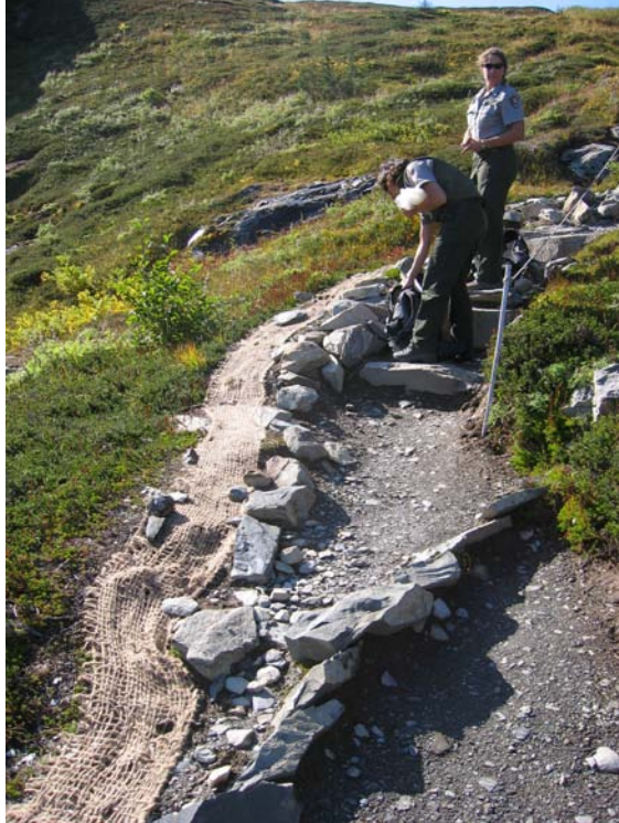
Biotechs Installing Jute Mesh. NPS Photo.
