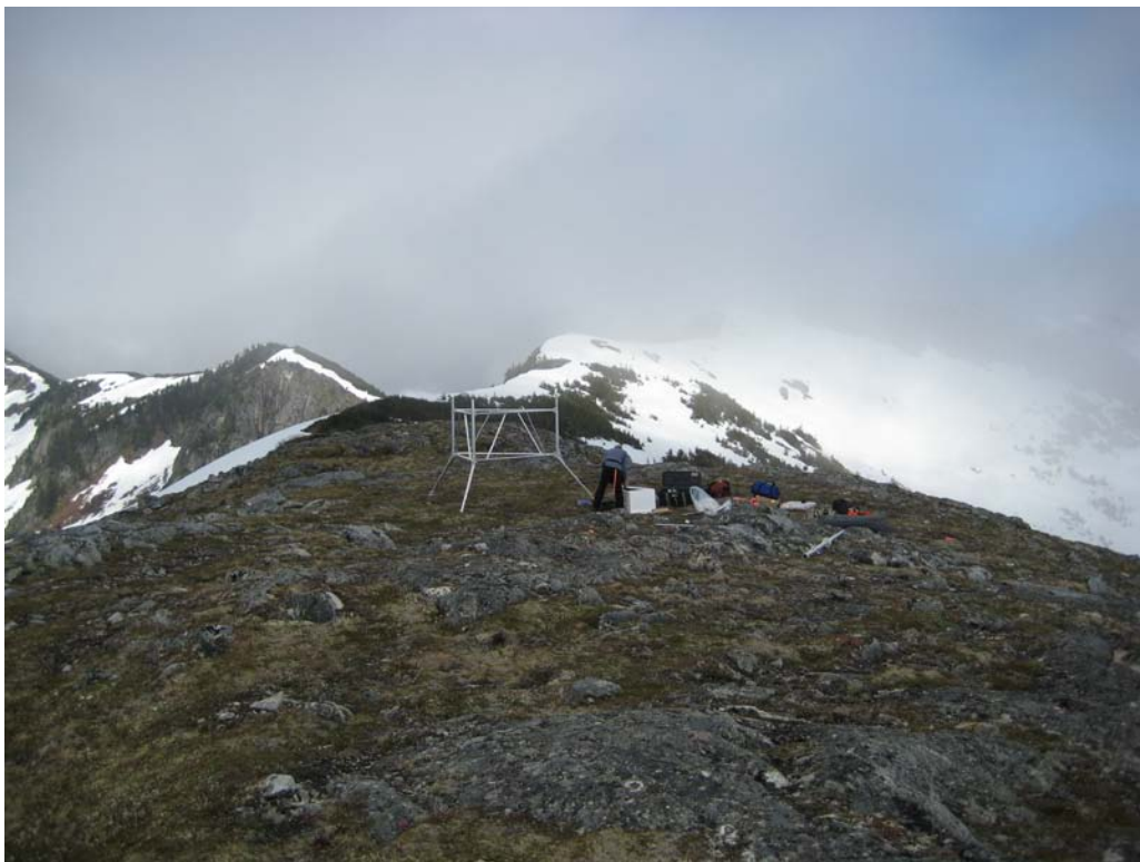
RAWS tower base in place. Note the footprint. 6/17/08
