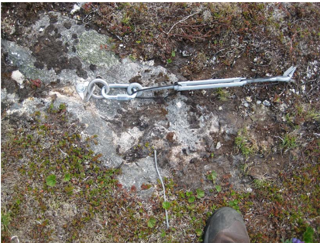
Expansion bolts anchored into bedrock. 7-02-08
