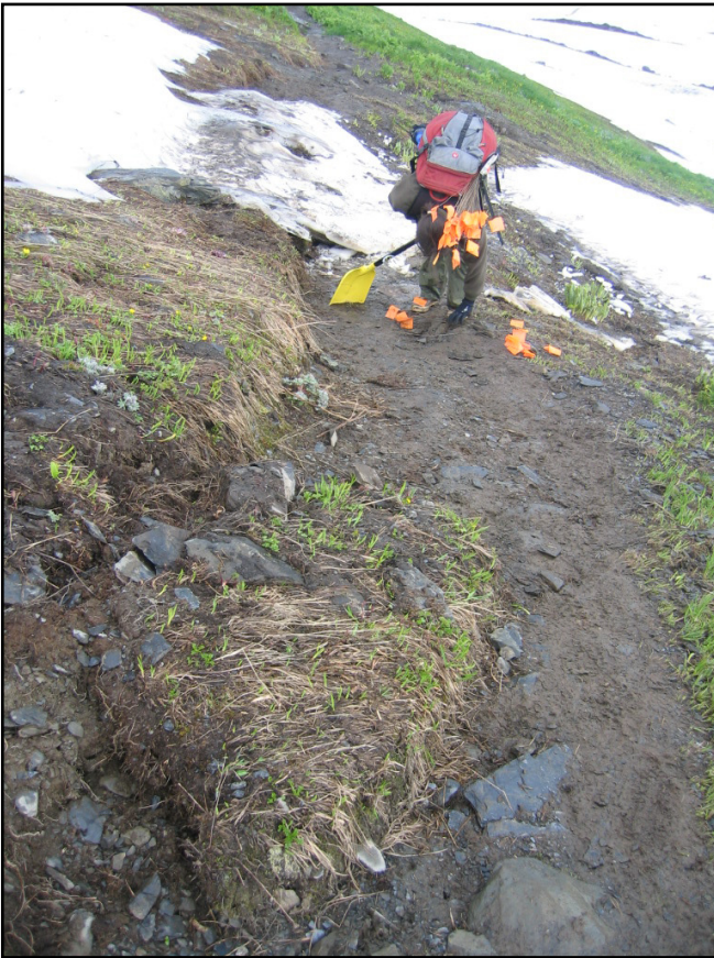
Figure 8. Saturated soils resulted in vegetation slumping onto the HIT beyond the Top of the Cliffs Overlook (mile 2.25). Photo taken 8/15/2008.
