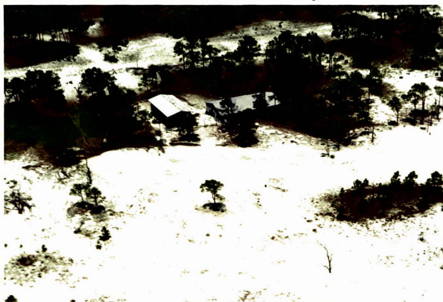
OUTSIDE WILDERNESS: BSF&W field station-cabin at left, corrugated metal storage building at right (6/7/71)
