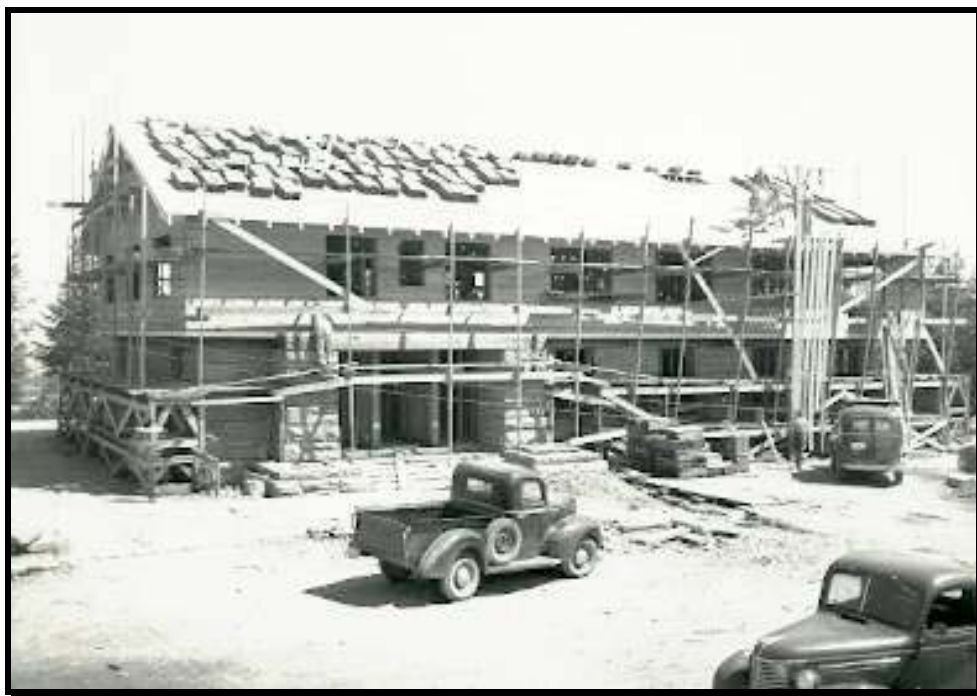
Figure No 1-1: Construction Progress, June 1940.
