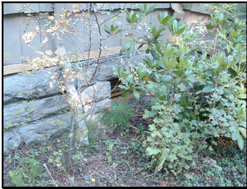
Figure No. 2-6: Existing foundation vent on rear elevation.
