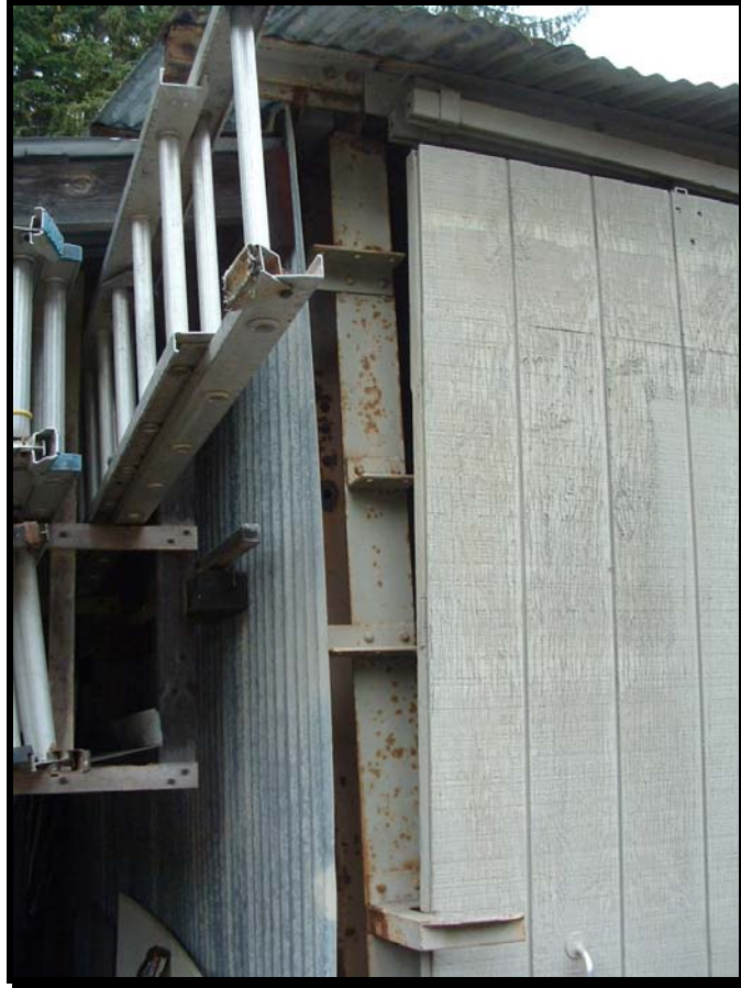
Figure No. 1292-3: View of southeast corner, November, 2009, showing the “I” beam column with original angle brackets
