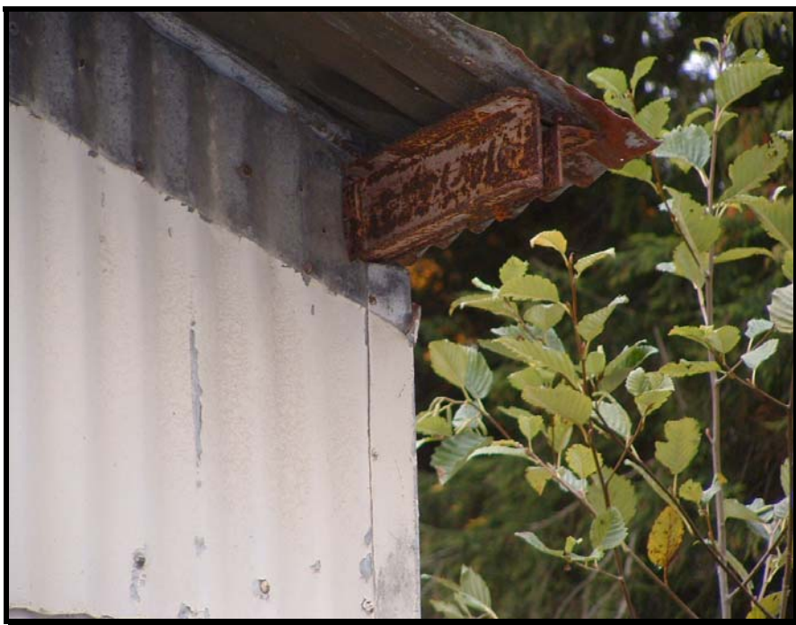
Figure No. 1292-4: View of northwest corner, November 2009, showing a channel purlin.
