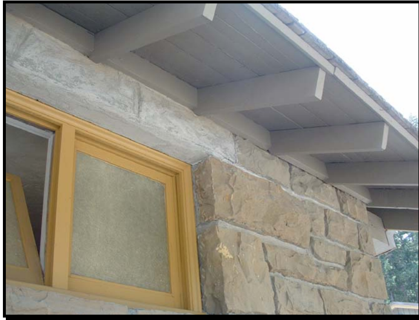
Figure No. 3-5: Note the faux stone plaster covered wood lintel above the window.
