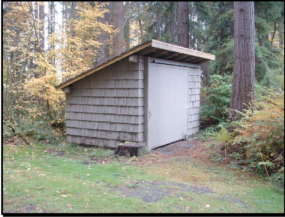
Figure No. 12-1: Superintendent's Woodshed, November 2009.
