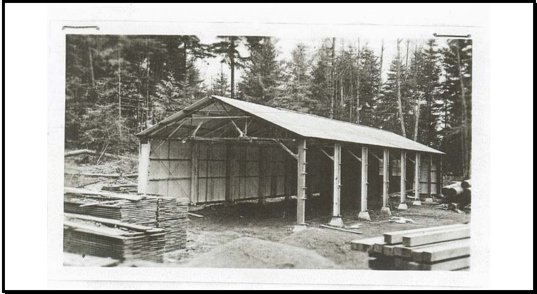
Figure No. 1292-1 This photograph is from the Superintendent's report of April 1956.
