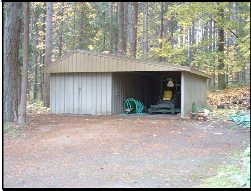
Figure No. 1240-1 View looking at the west elevation, November 2009.
