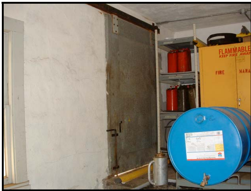
Figure No. 3-7: Kalamien fore door at loading dock.
