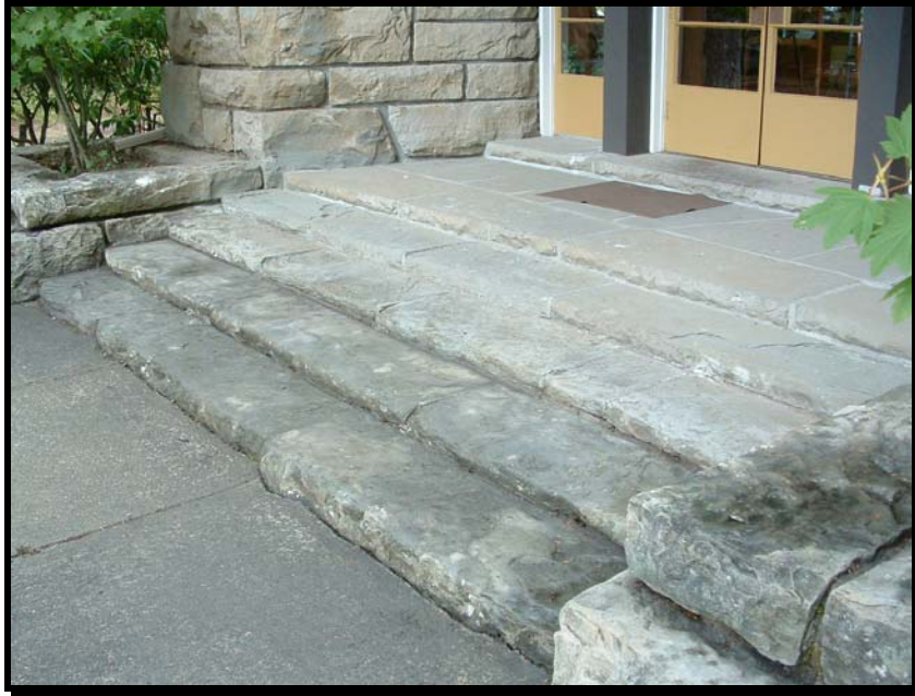
Figure No. 1-12: Front entry steps and landing.
