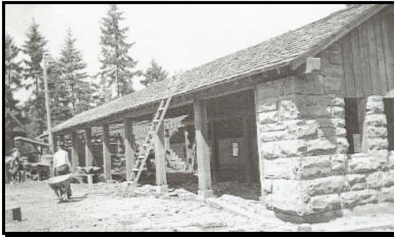
Figure No. 5-1: Equipment Shed under construction, spring 1941.
