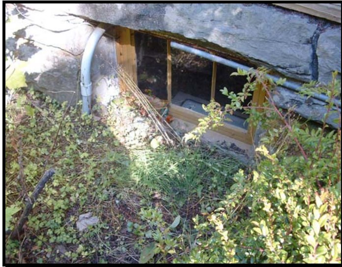
Figure No. 2-8: Shallow window well
