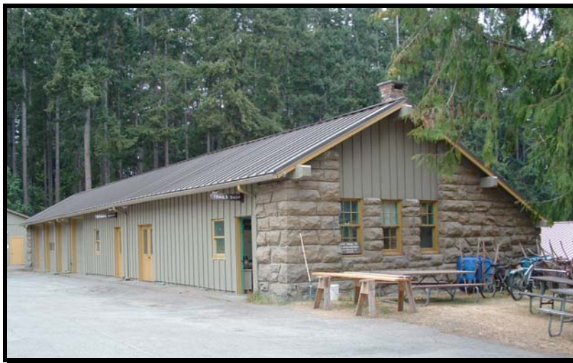
Figure No. 5-2: Equipment Shed, August 2009.
