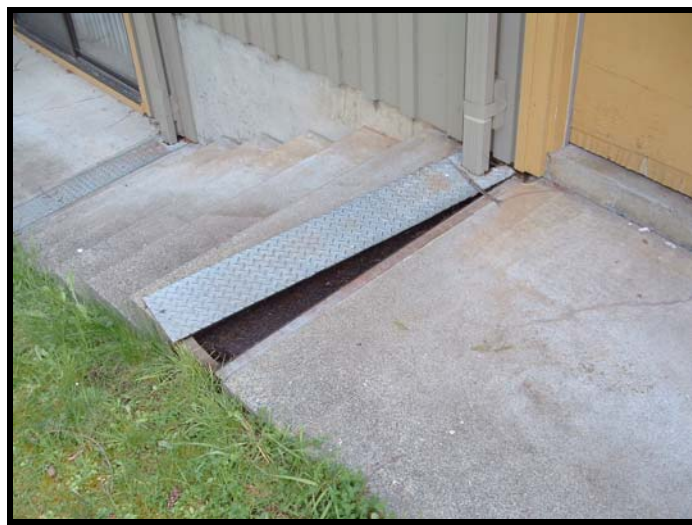
Figure No. 17-2: Drain troughs for rear elevation downspouts.
