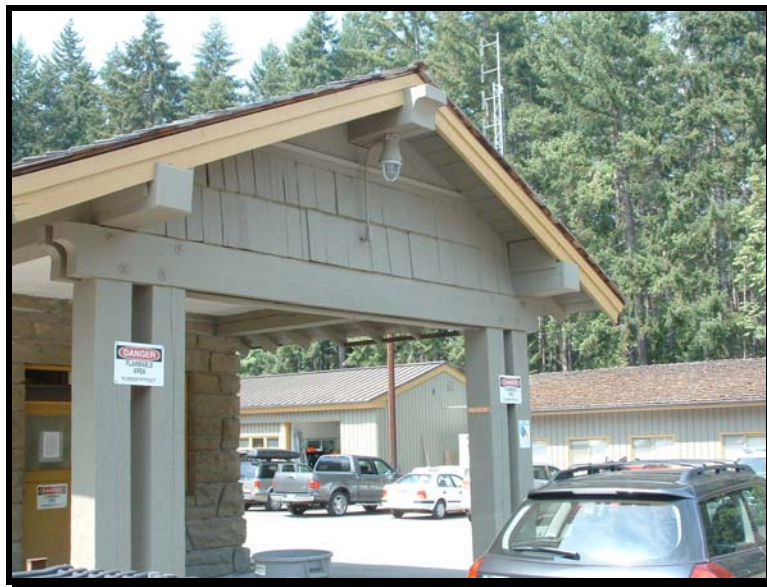
Figure No. 3-6: Note the cavetto profiles on the ridge outlooker and cross girders.
