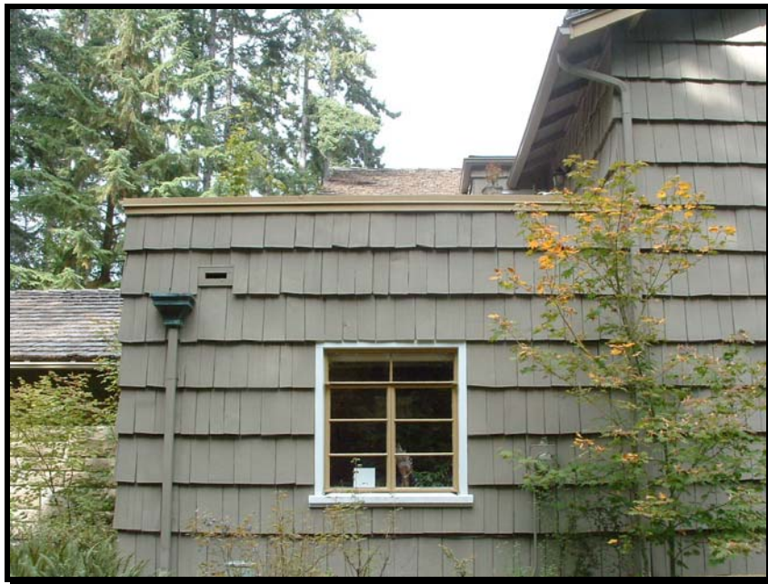
Figure No. 2-16: The drain from the sundeck discharges into the leaderbox; the opening to the right of the leaderbox is the overflow scupper.
