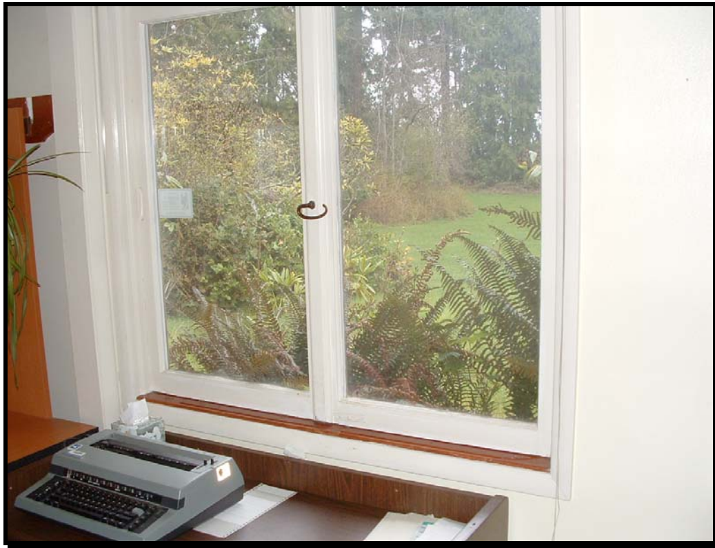
Figure No. 20-3: Offset horizontal slider windows; note groove in the windowsill.
