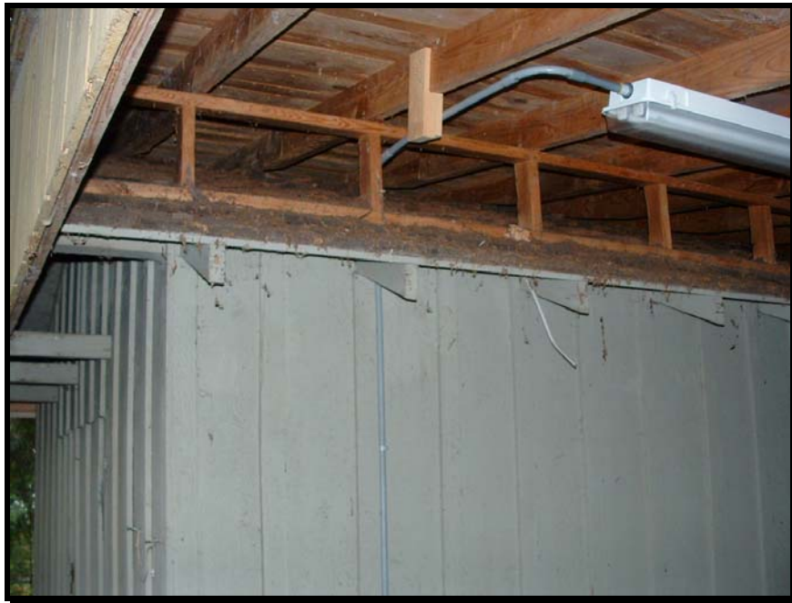
Figure No. 1240-2 View of short "pony wall" located above the sidewall of the original wall below; the original shingle roof is still visible, November 2009.
