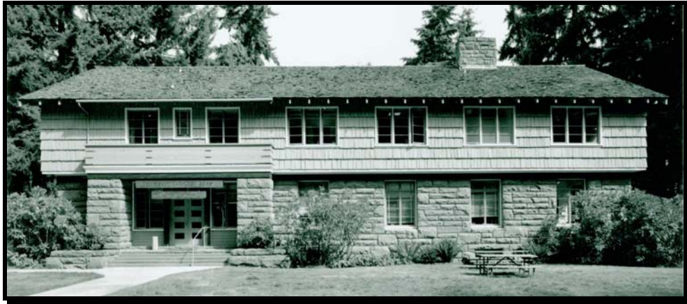
Figure No. 1-5: Administration Building, 1983; note lack of gutters and downspouts except over entry.
