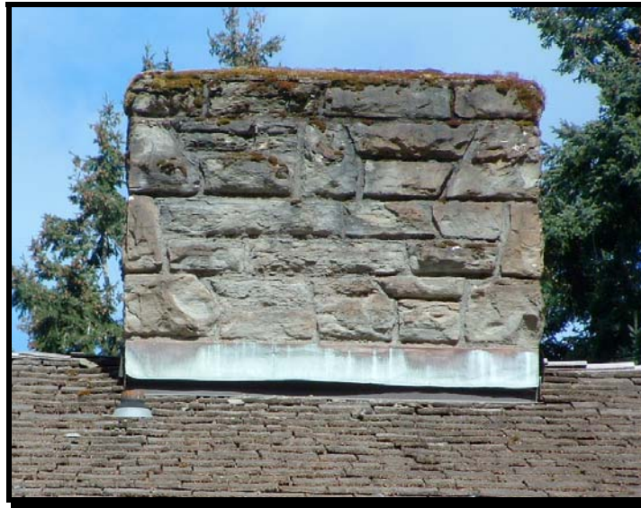
Figure No. 1-10:North side of the chimney
