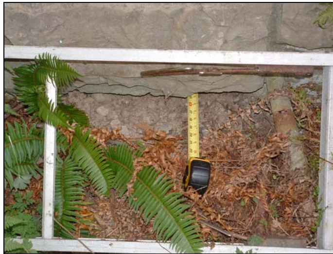
Figure No. 4-4: Opening through stone foundation to under interior floor slab.
