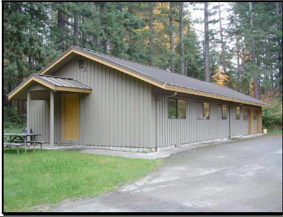
Figure No. 16-1:BRD Offices (former apartment garage), November 2009.
