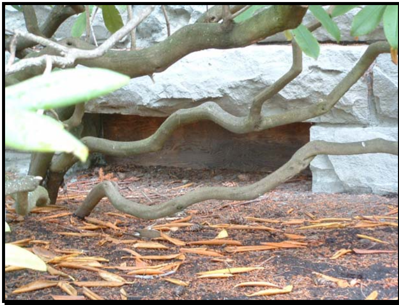
Figure No. 1-7: Foundation vent.
