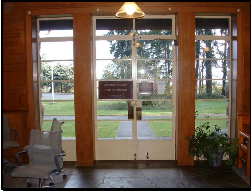
Figure No. 1-14: Steel front entry doors
