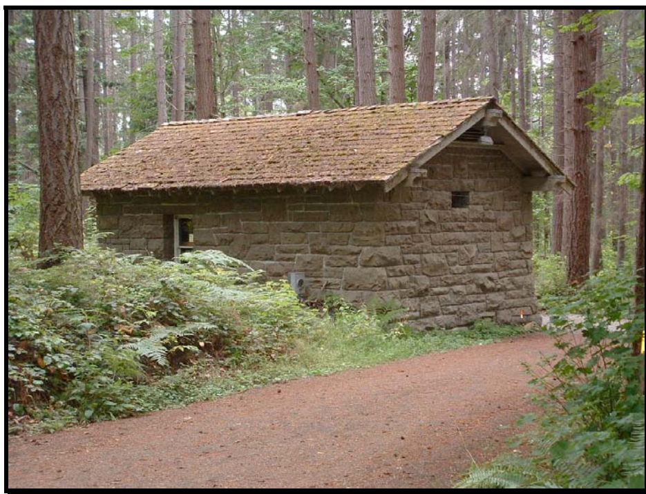
Figure No. 4-2:Transformer and Pumphouse Building, August 2009.
