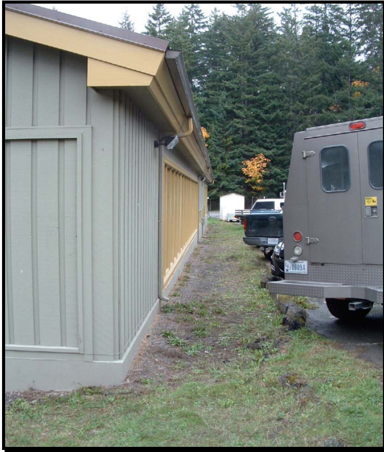
Figure No. 9-3: The uphill side of the building captures both the drainage of the parking area and the roof drainage.
