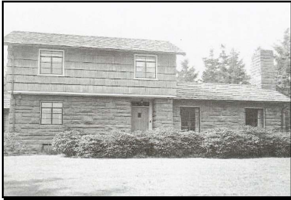
Figure No. 2-5: View of north elevation, 1943, less than two year after Superintendent Macy and his family moved into the completed building.
