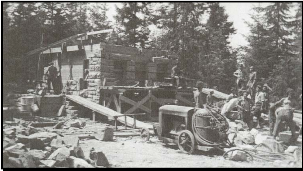
Figure No. 3-1: Gas & Oil House under construction, June 24, 1940.
