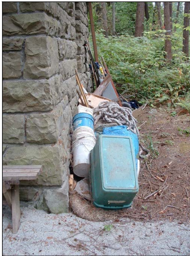
Figure No. 4-3: Equipment and tools stored against the west wall.
