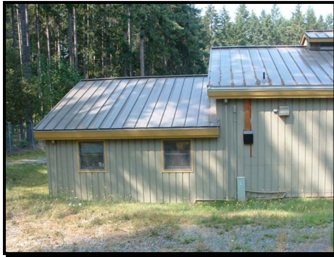
Figure No. 1000-6: Unpainted siding repair at southwest corner.
