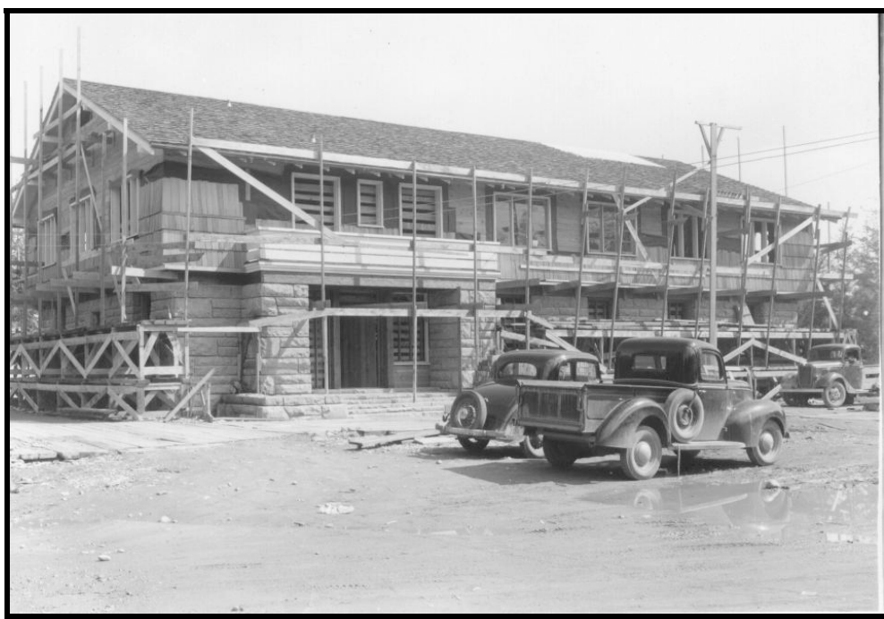
Figure No. 1-2: Construction progress, July 1940; from Superintendent's monthly report of August 10, 1940; construction halted at this point until February 1941.
