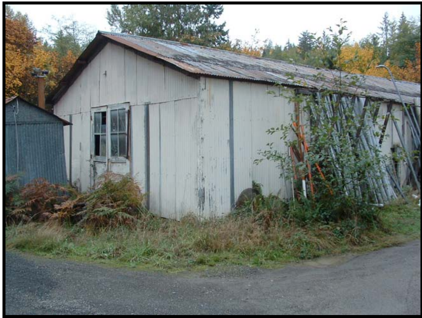
Figure No. 1292-2: View of northwest corner, November 2009.
