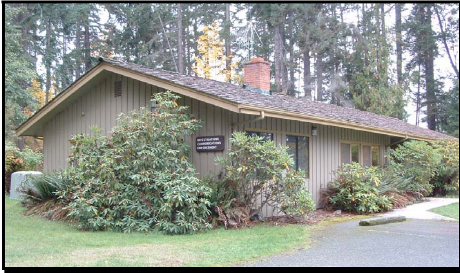
Figure No. 20-2: Original Assistant Superintendent's house; now used to house law enforcement investigations, communications, and enforcement, i.e. "Ice House".
