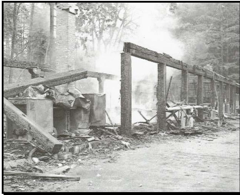
Figure No. 1000-2: Fire damage of 1965.
