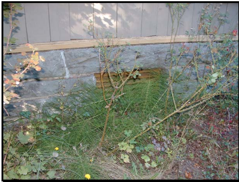
Figure No. 2-11: Note the trim moldings atop the stone
