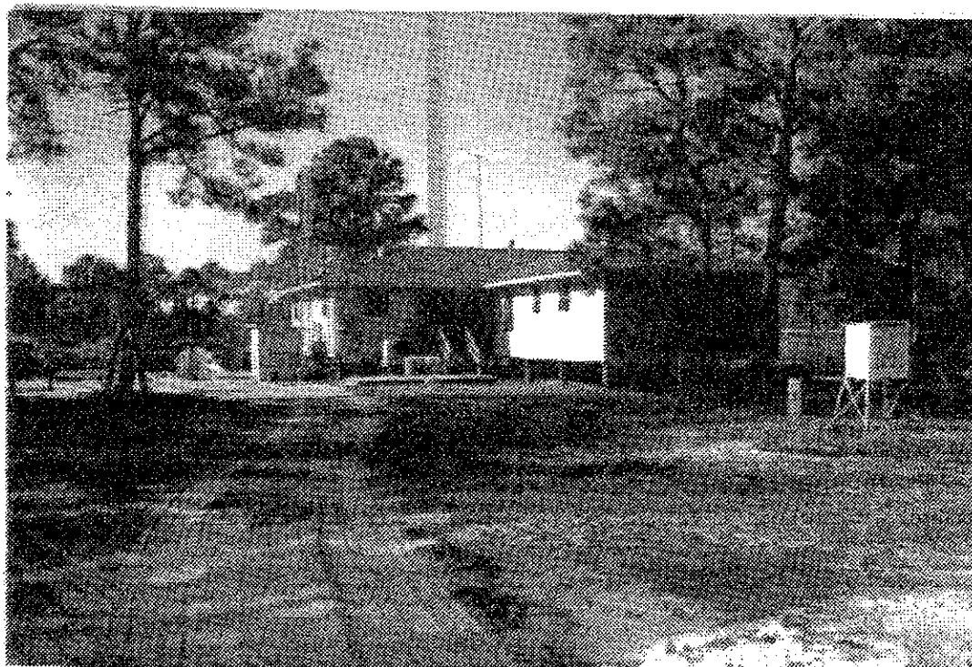
HORN ISLAND Quarters 31A, B, C Overall View November 8, 1994
