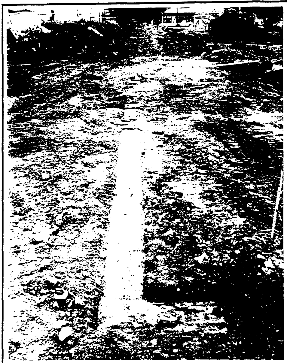
Figure 62. East wall foundation of the Thibodeaux Boiler Works Co., Ltd. (27 June 1989). View is to the south.
