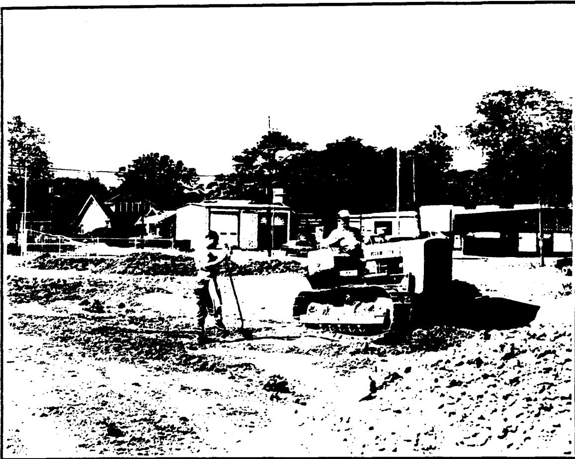
Figure 48. Stripping of Strip Area 2, Strip Area 1 is in the background (6 May 1989). View is to the southwest.
