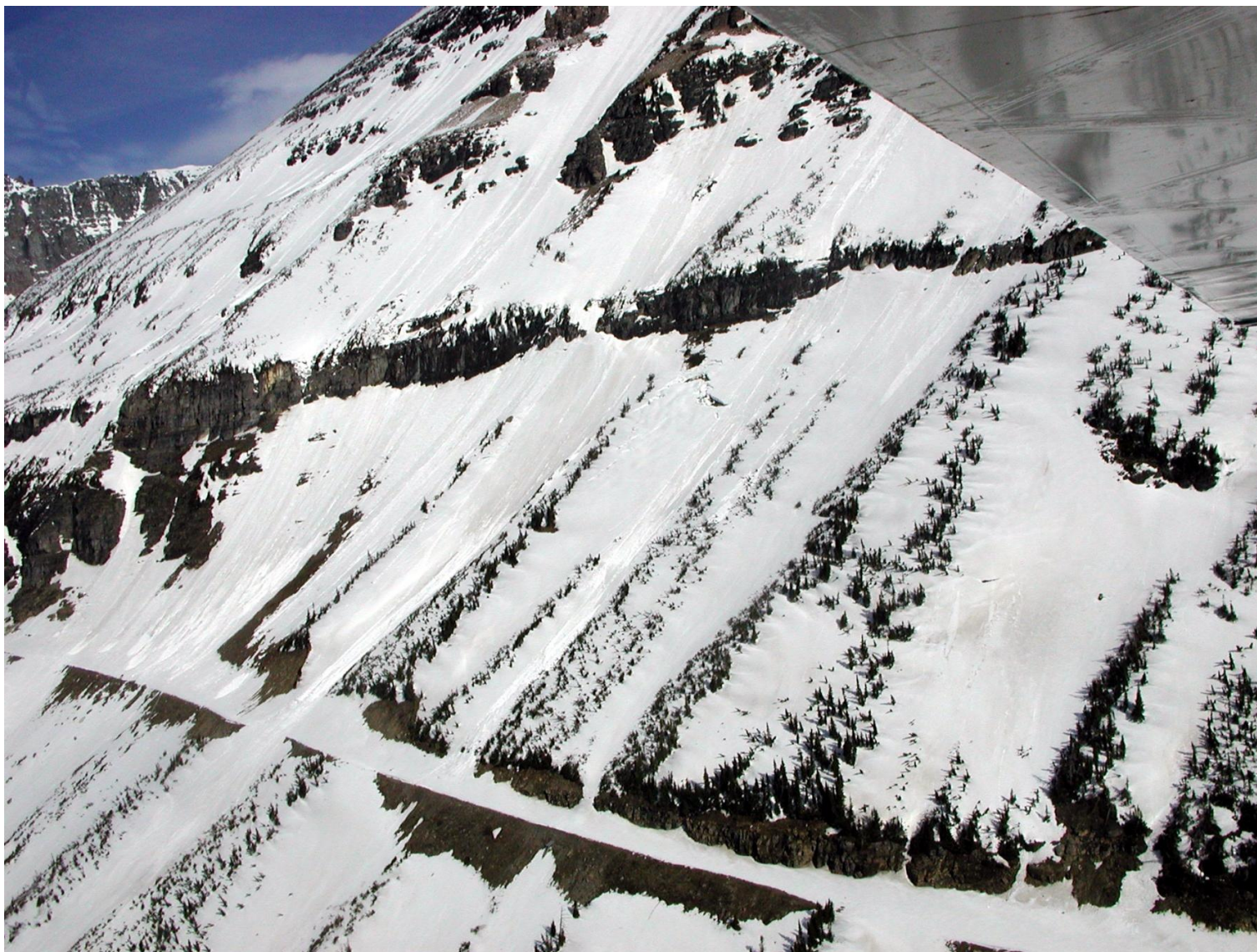
1 / 51 Slopes Below East Tunnel
