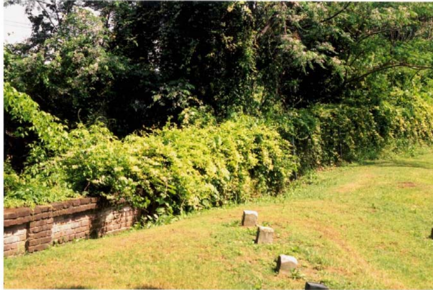
Figure 3 Northwest Wall with Excessive Vegetation Growth
