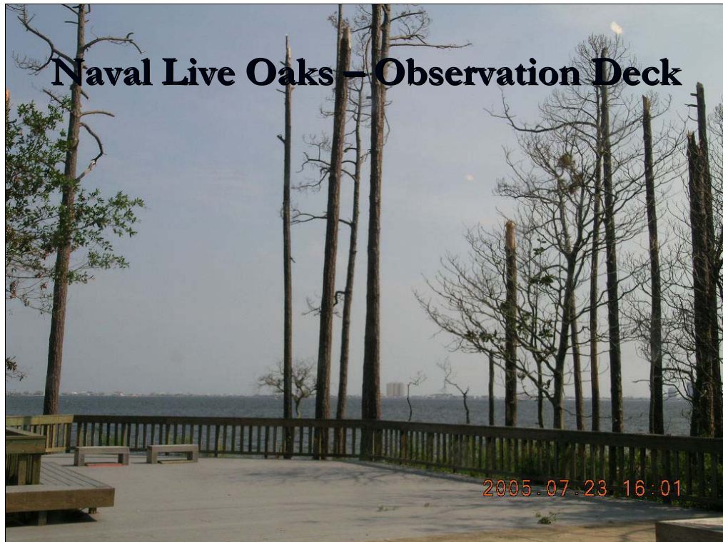
July 23 - Observation Deck behind the Naval Live Oaks visitor center after crews removed hazard snags and the area had reopened to the public.
