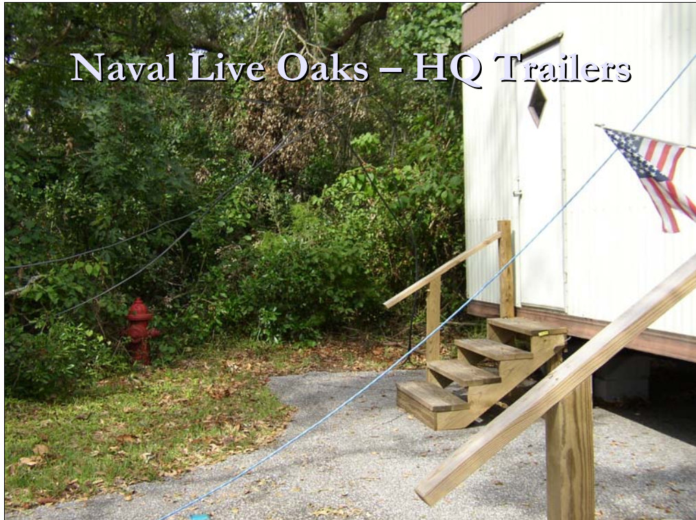
July 19 – Temporary power lines strung between park headquarters and park offices in trailers nearby.
