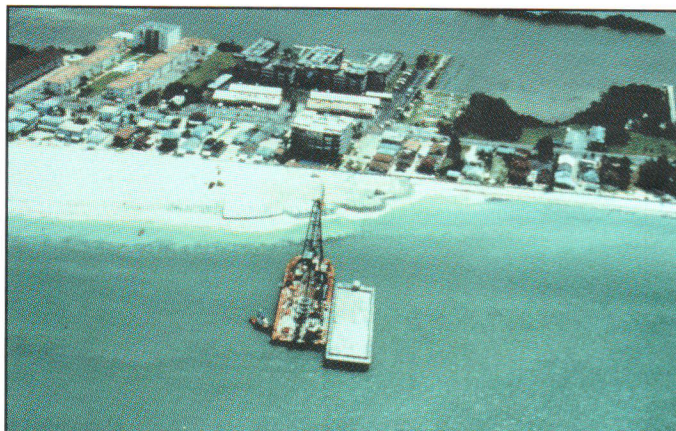
A recent beach nourishment project at Sand Key is an increasingly common countermeasure to beach erosion in highly developed coastal regions.
