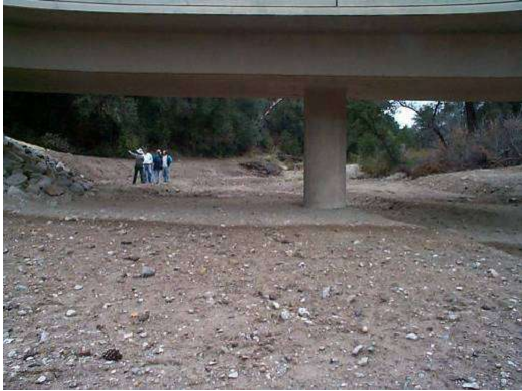
Figure 6. Chalone Creek, Pinnacles NM, under summer baseflow conditions, and prior to growth of vegetation in channel.
