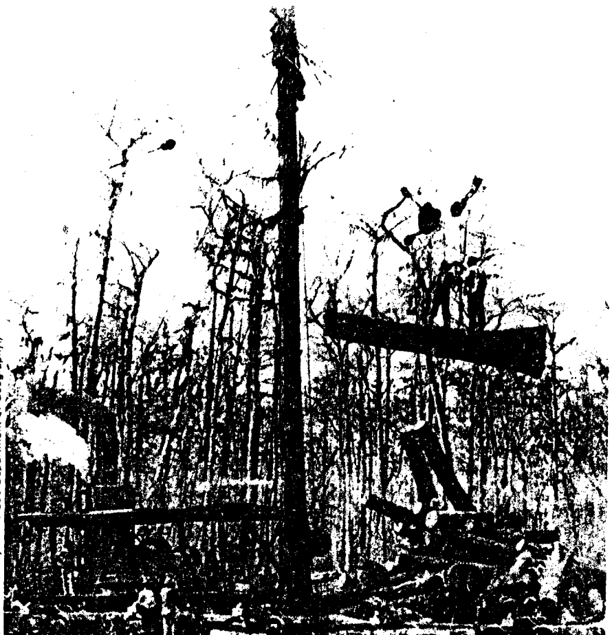
Steam-powered skidders with overhead cableways were a major innovation to the baldcypress logging industry in the late 1800s.
