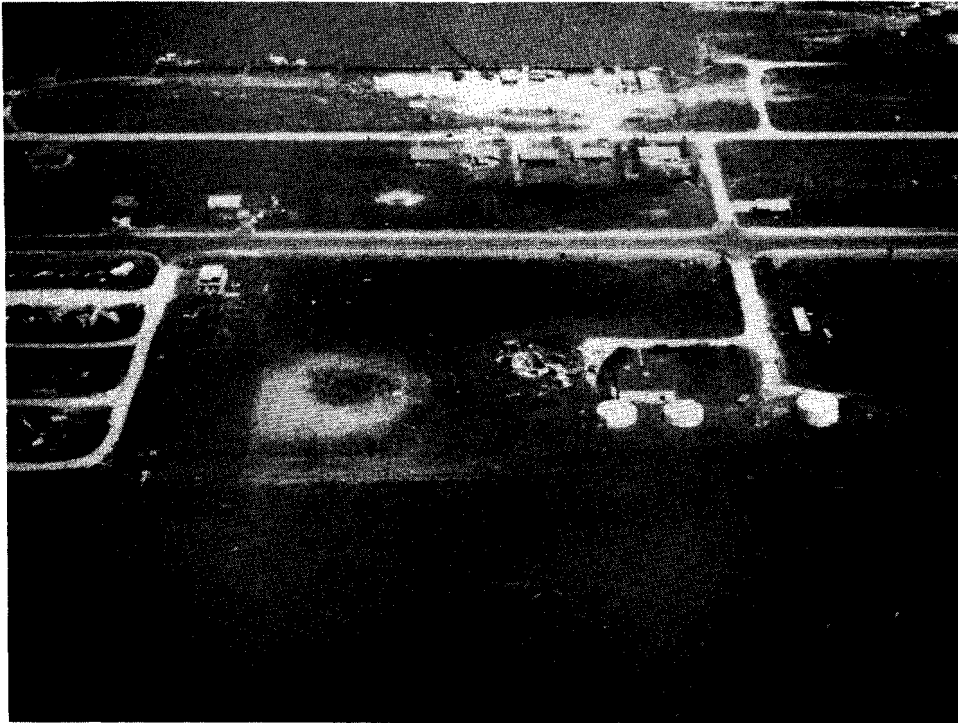
Industrial Damage - Port Mansfield
