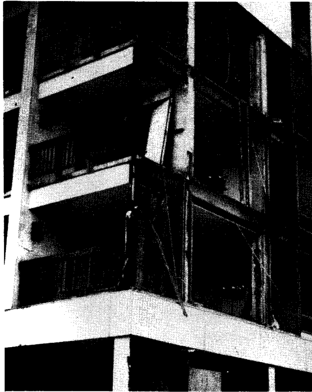
Commercial Damage - North Padre Island
