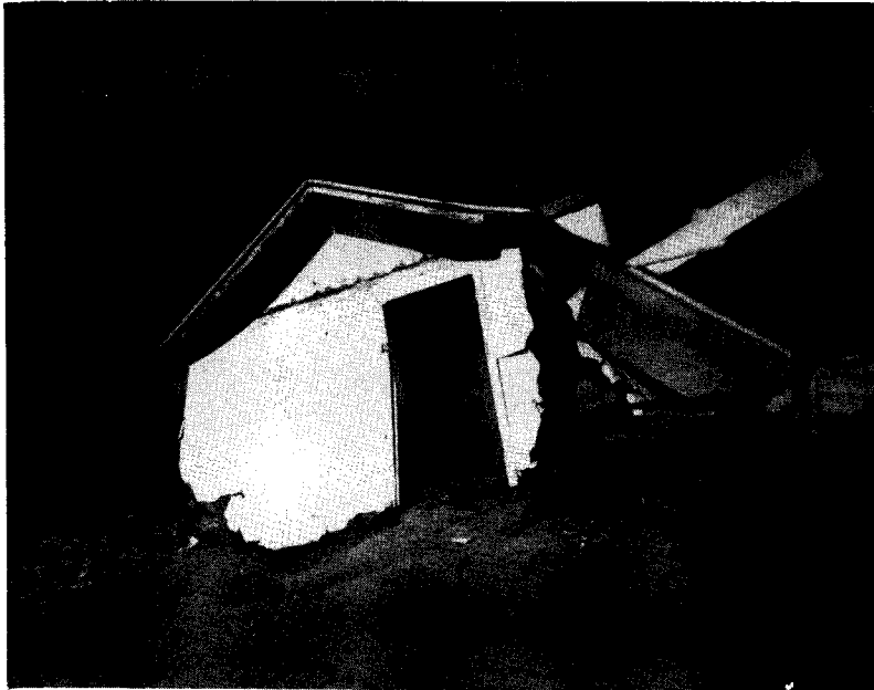
Residential Damage - Port Isabel
