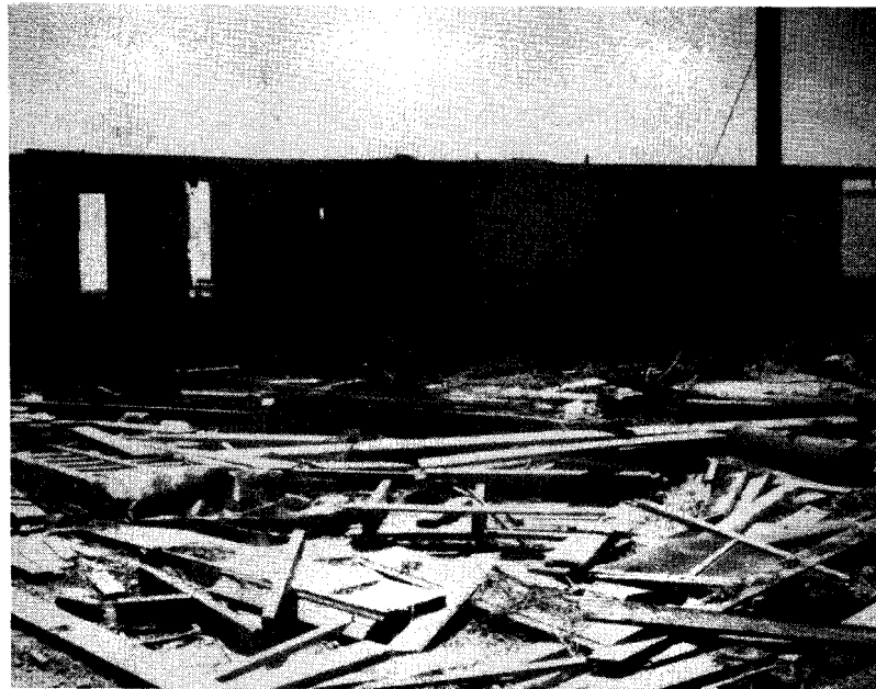
Commercial Damage - Port Mansfield
