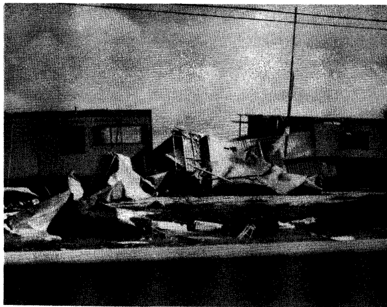
Residential Damage - Port Mansfield
