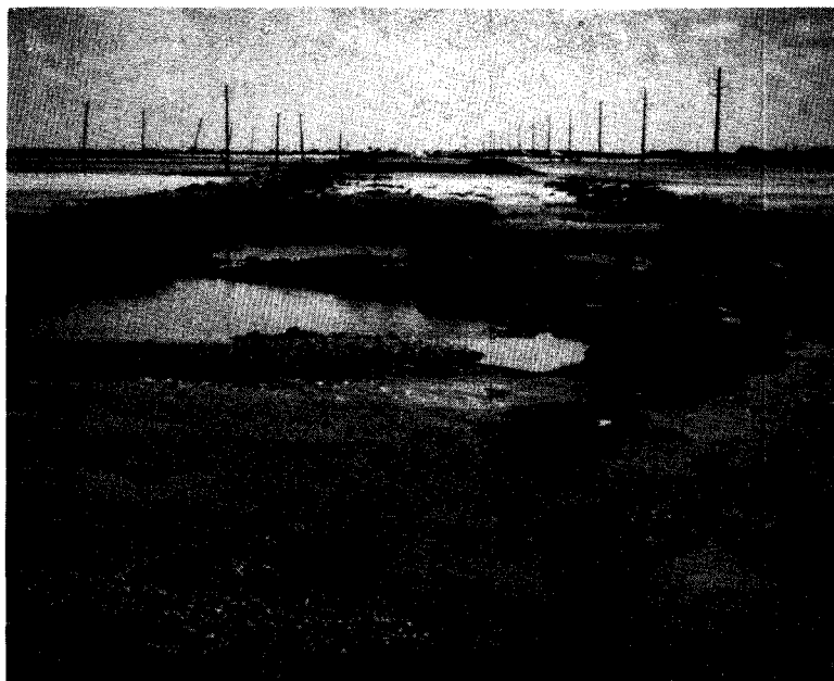
Road Damage - Mustang Island
