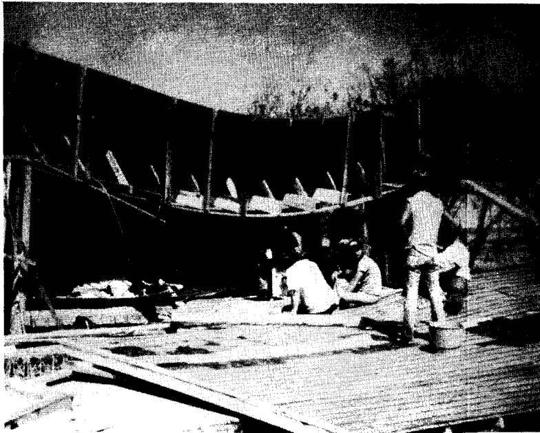
Residential Damage - Port Mansfield
