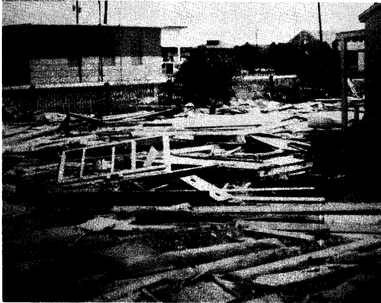
Residential Damage - Arroyo City
