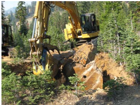
Removing one of several underground septic tanks at Sulphur Works
