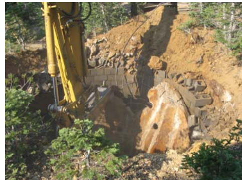
Removing one of several underground septic tanks at Sulphur Works
