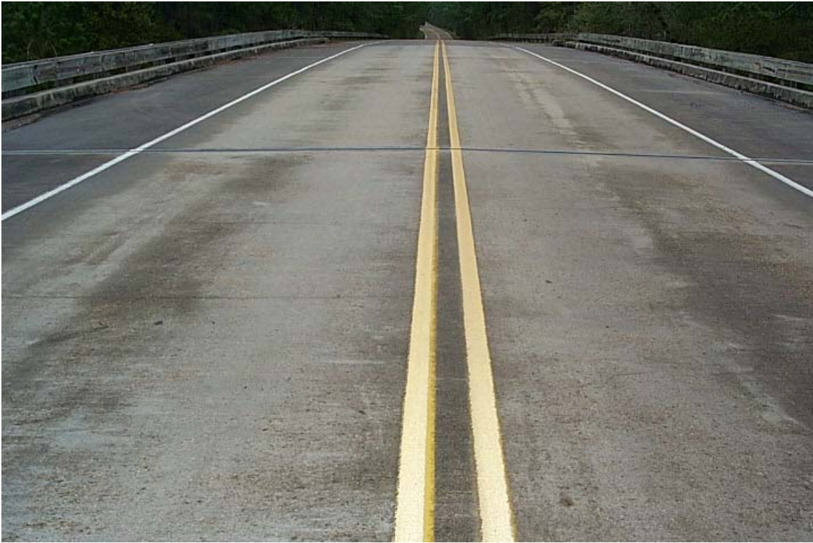
PHOTO #1 - GENERAL VIEW OF DECK (PHOTO FROM 3/20/01 INSPECTION REPORT)
