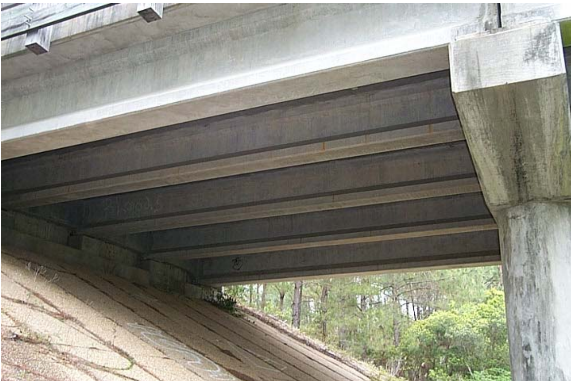
PHOTO #2 - UNDERVIEW OF NORTH SPAN
