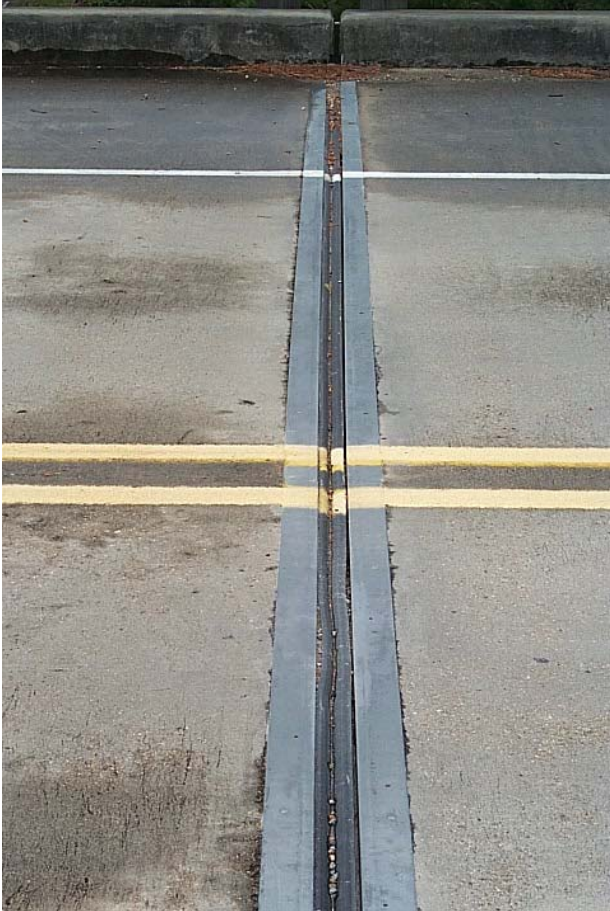
PHOTO #3 - EXPANSION JOINT AT NORTH PIER (PHOTO FROM 3/20/01 INSPECTION REPORT)
