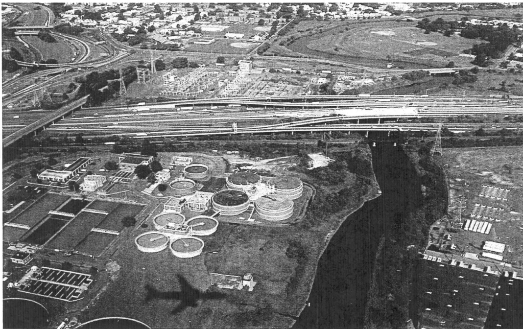
Sewage Treatment Plant
