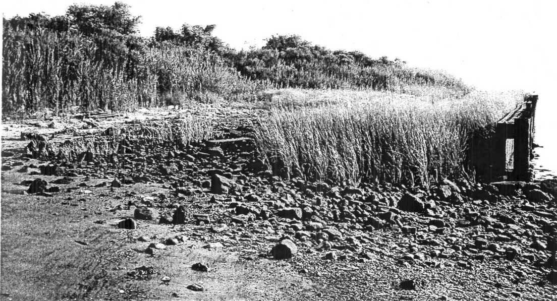
Figure 11. The backshore area behind the wooden bulkhead is tide dominated. Because the bulkhead maintains an elevated terrain behind it, Spartina is able to grow along the edges of the small tidal pools created by the bulkhead.
