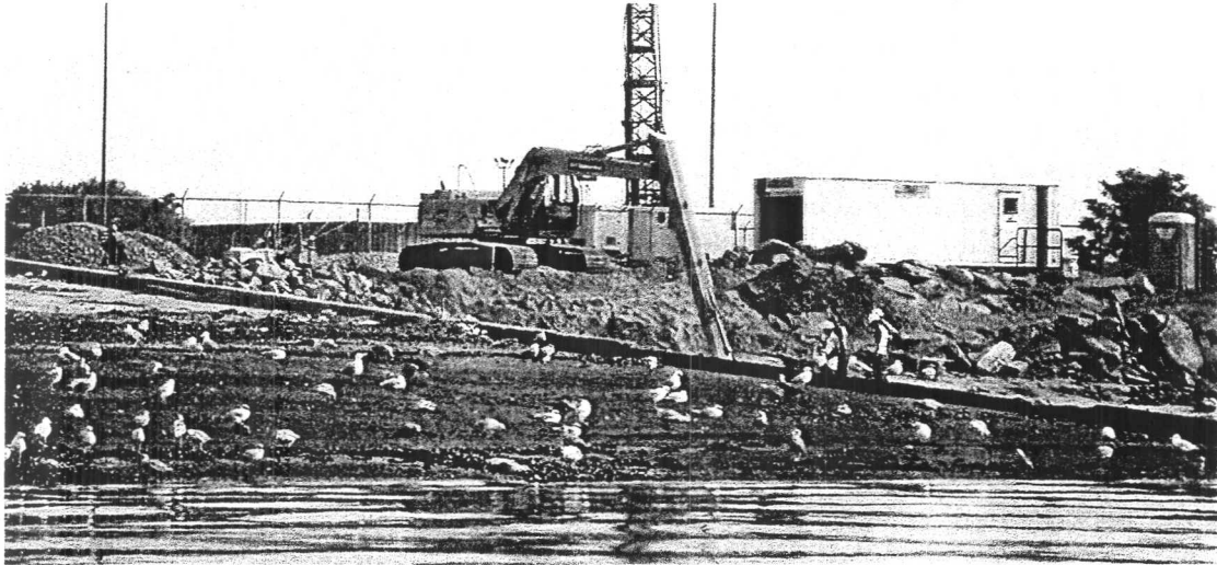
Figure 4. Emplacement of armor stone on the graded slope is underlain by filter cloth to prevent sediment washout through the armor stone face.
