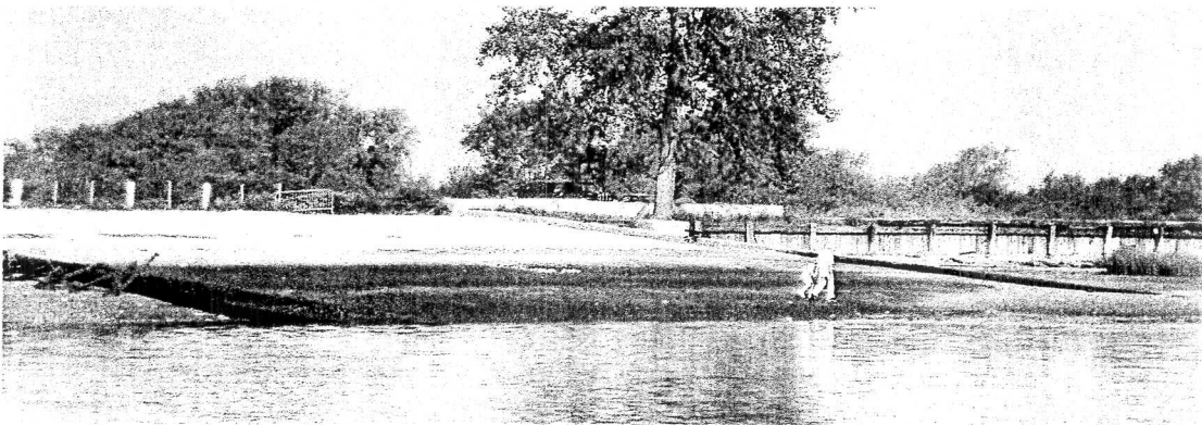
Figure 8. Looking north past the Hangar B seaplane ramp. Note the wooden bulkhead on the backshore. Sediment has accreted on the south side of the ramp indicating that longshore sediment drift is predominantly northward. Sediment accretion on the north side of the ramp is from the drainage culvert source.
