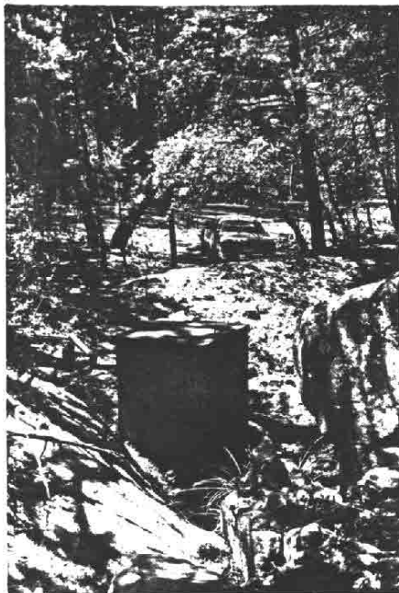
Chiricahua, Shake Spring, looking South. The box (below center) sits above the collection basin for Shake Springs. Access to collection basin is by means of circular opening in floor of box. The GSA vehicle (above center) sits backed off of park road.
