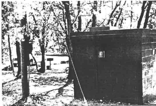
Chiricahua, Campground Well, looking South. This well is located in this pumphouse (back view) located within campground area of park. GSA vehicle is parked at a turnout for one of the campsites.
