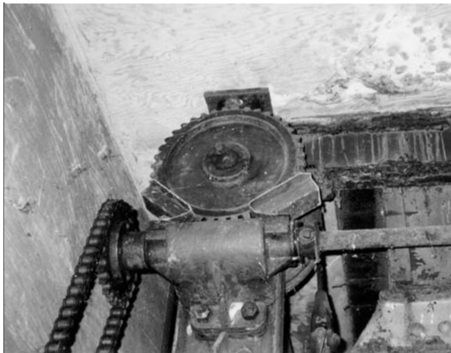
Figure 9. Interior view of the elevator platform operating mechanism.
