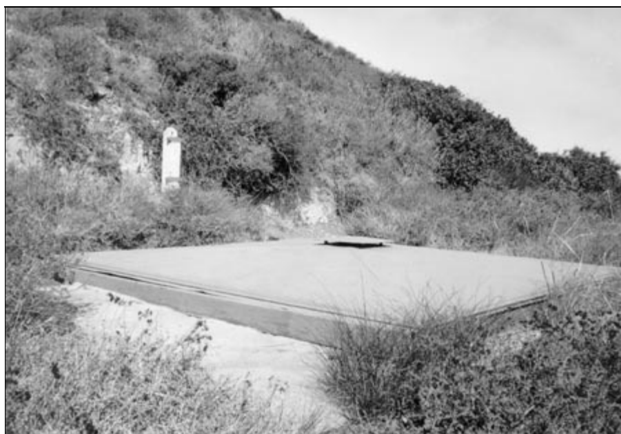
Figure 12. Only the metal roofs and a concrete post are visible above ground.
