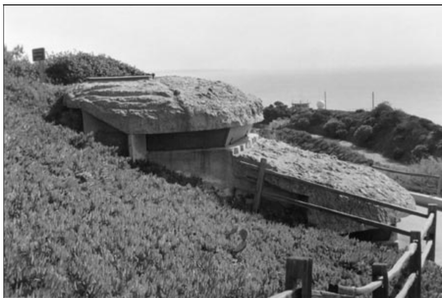
Figure 22. Battery commander station and base-end station, Battery Humphreys. Rough-textured concrete roofs provide camouflage for these structures.
