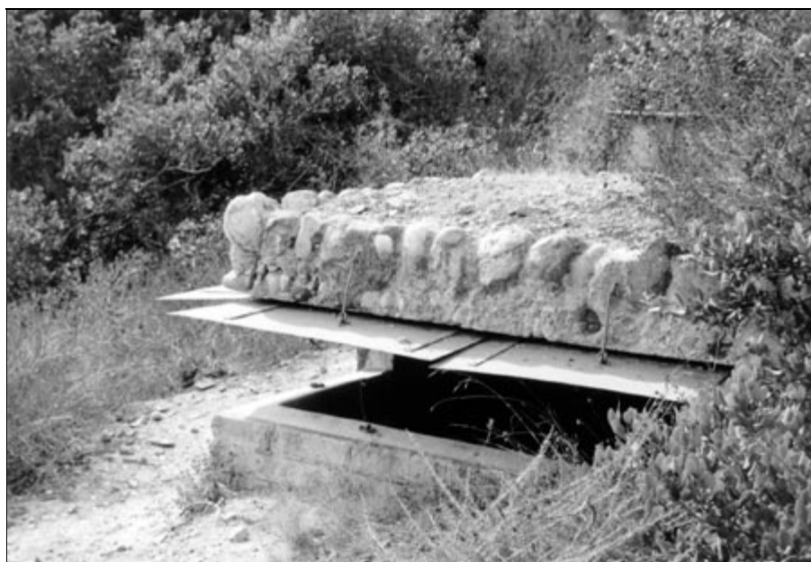
Figure 18. Metal shutters in the open position allow visual access through observation slots.
