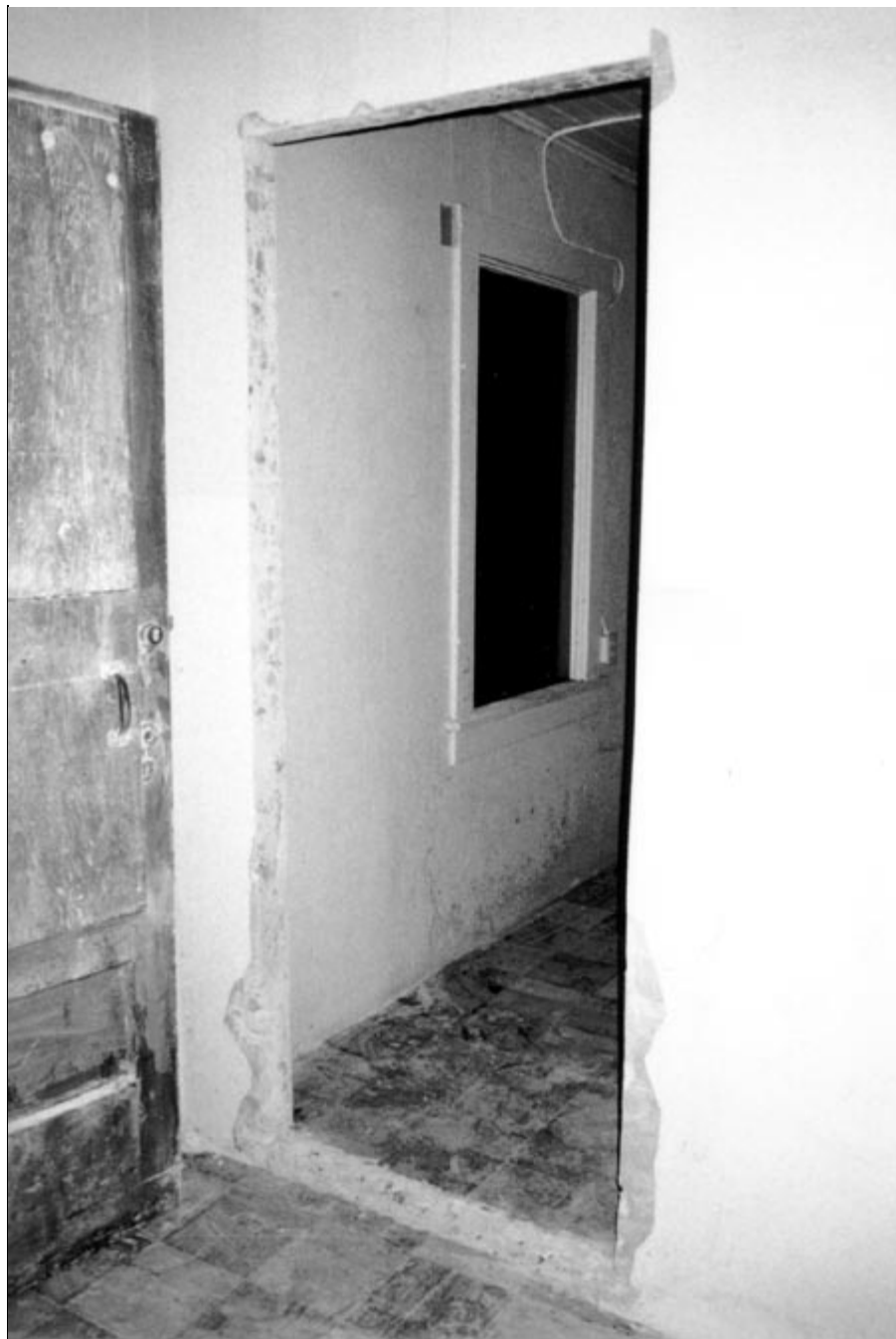
Figure 6. A non-original opening connects the Operating and Motor Generator Rooms.
