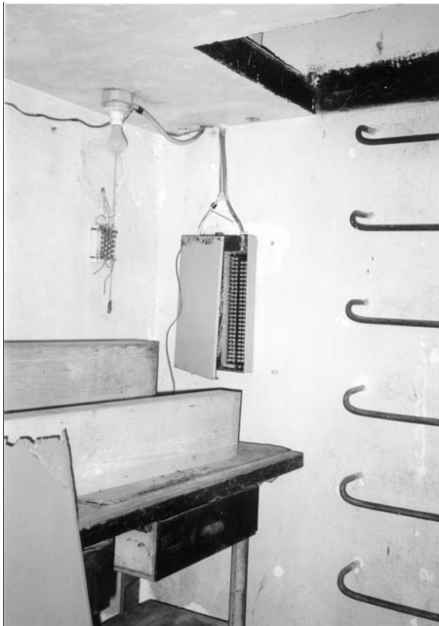
Figure 25. Embedded metal ladder rungs provide access to both floors of Ashburn's base-end station.
