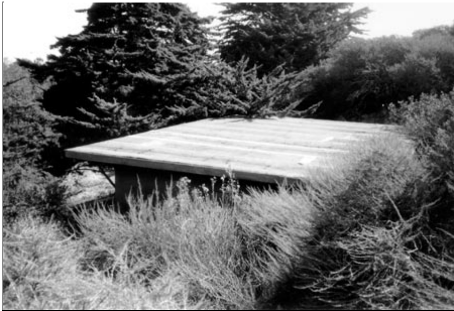
Figure 5. Roll-roofing clads the roof of the Army Radio Station.
