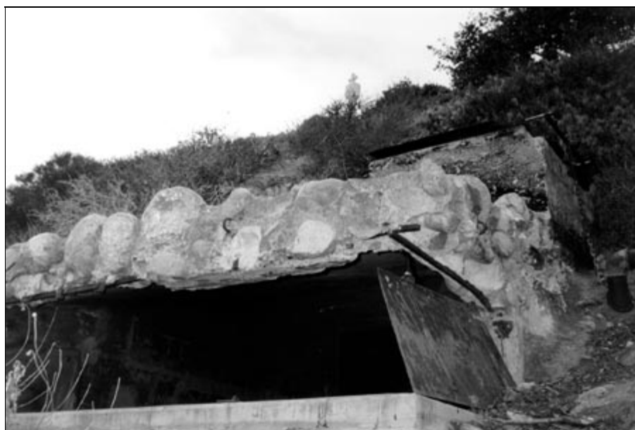
Figure 16. The missing metal observation slot shutters are located inside this structure.
