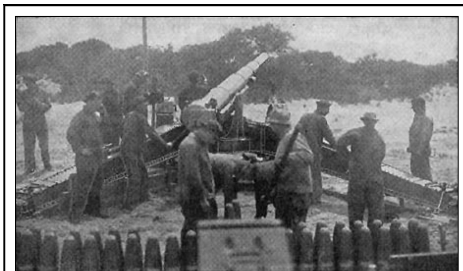
Figure 2. Battery Point Loma once featured 155 mm guns mounted on field carriages.
