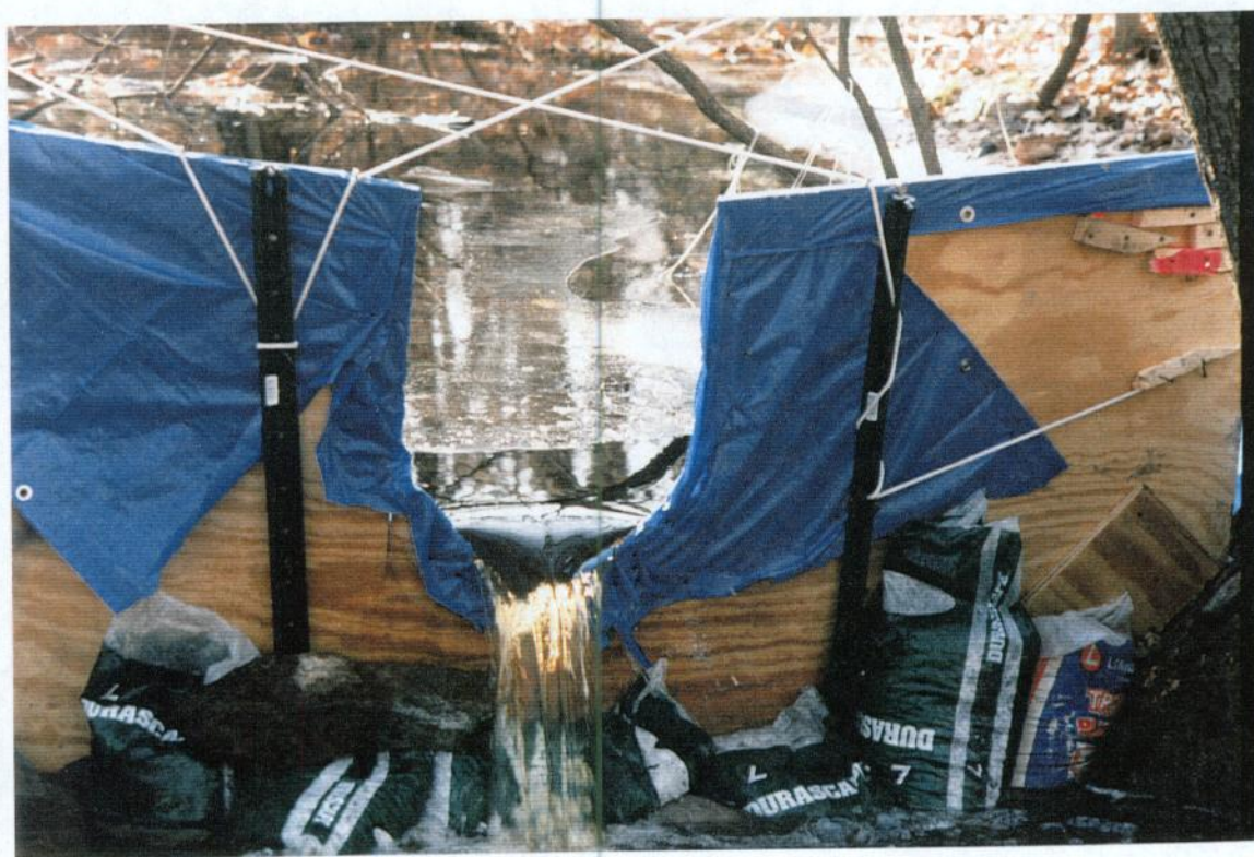
Plates 4 and 5: The 90 degree, v-notch weir was placed at the north end of the Bog to measure discharge. It was constructed of treated, exterior plywood and was stabilized with posts, rope, sandbags, and rocks.
