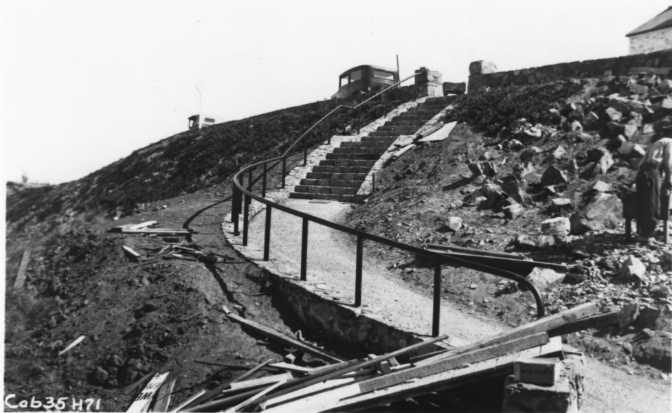
CAB35H71 West entrance steps to comfort station after installation of hand rails, bitumuls walks and boulders on highway guard wall.
