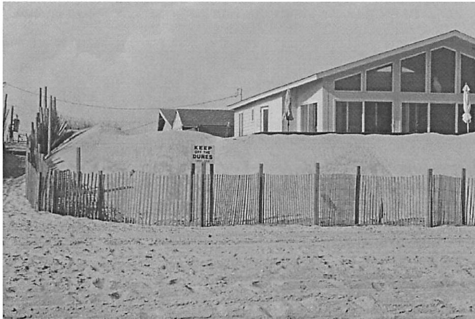
Figure 11. Beach scraping to create artificial dunes for erosion mitigation is a common practice in the communities on Fire Island. Snow fencing is generally used in conjunction with scraping to help hold the sand in place.
