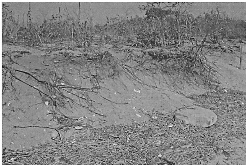
Figure 15. Erosion of artificial sand levees around West Pond in Jamaica Bay.
