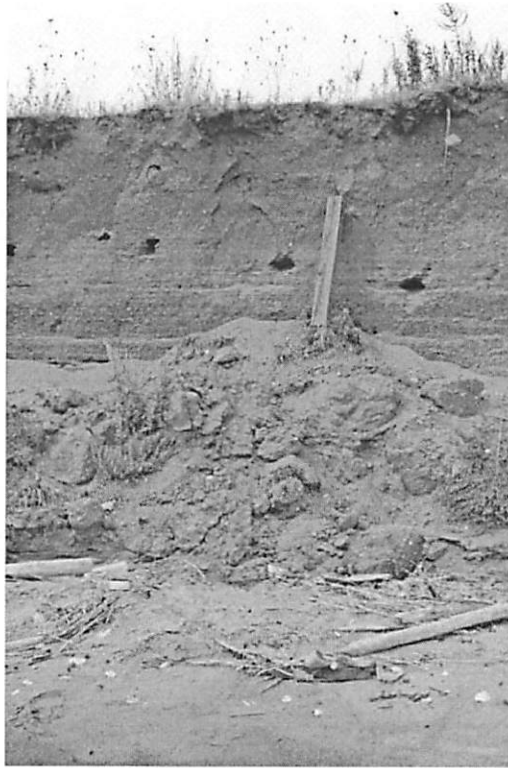
Figure 17. Rapid erosion of bluffs composed of soft glacial outwash deposits is threatening a bathhouse in Great Kills Park.
