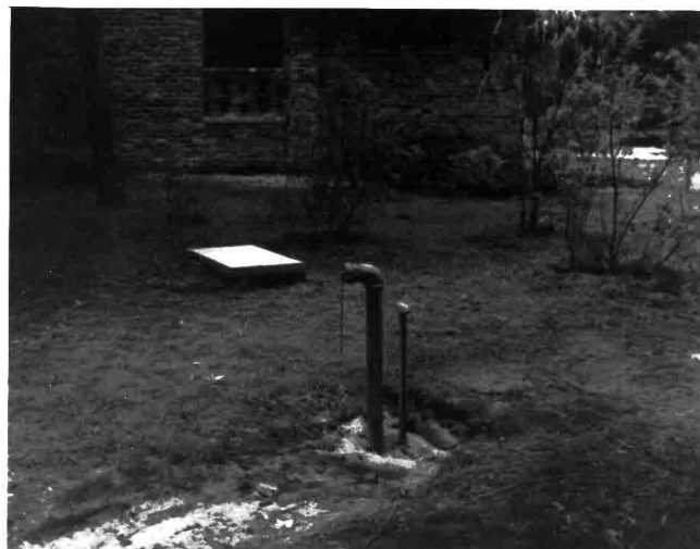
WELL (UNDER CONCRETE SLAB)
