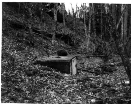
SPRING ENCLOSURE AND INTAKE
