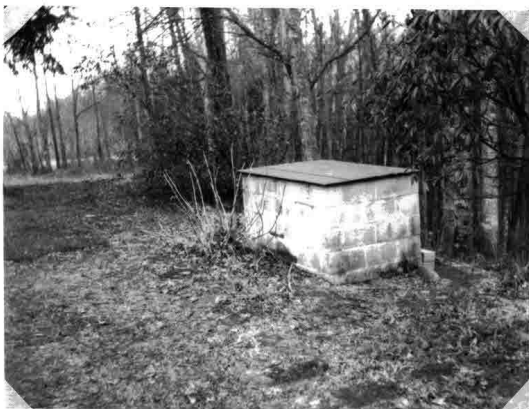
PUMP HOUSE AT RESIDENCE
