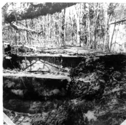
15,000 Gallon Concrete Reservoir and Chlorinator House Serving Balsam Mountain Campground
