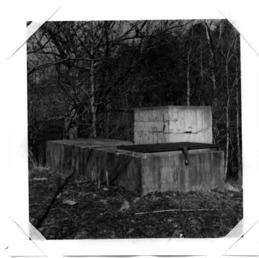
Existing 2,000 Gallon Concrete Reservoir Serving Cable Mill Area
