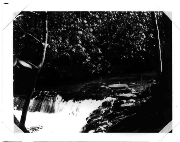
DAM AND INTAKE STRUCTURE
